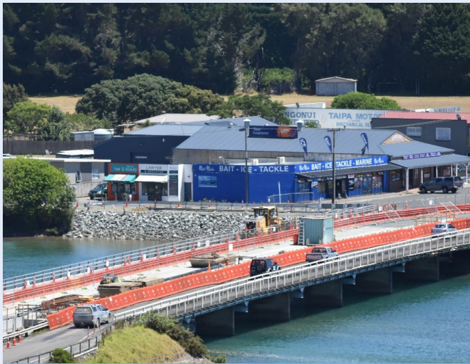
Final day of traffic on the old bridge - 14 February 2019.
