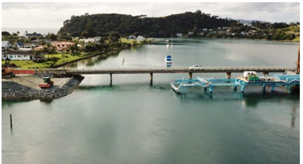
Looking northwards down Taipā River. The visible sloped concrete at the top of the rocks on the township side causeway is called an abutment and this is where the bridge is connected to the causeway.
