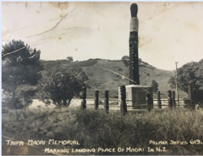
The original Taipā Māori Memorial/ Pouwhenua that blew over in a cyclone.
