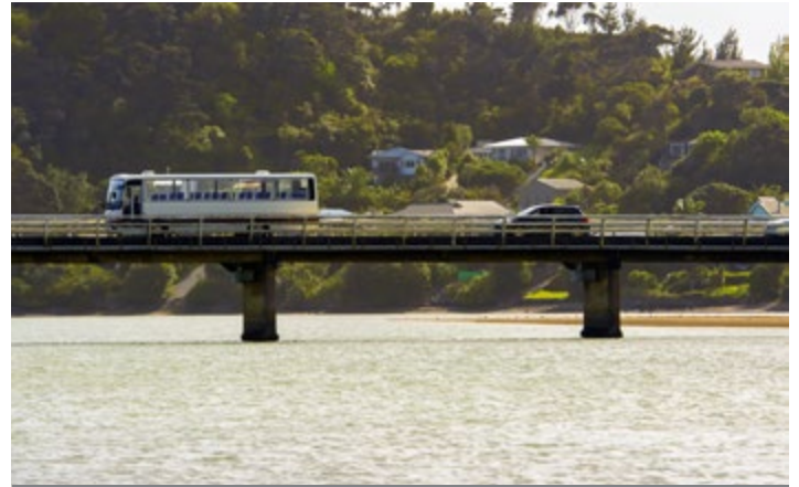
Taipā's existing single lane bridge has six piers in the waterway compared to the new bridge which will have only three piers in the waterway. Photo: Malcolm Pullman
