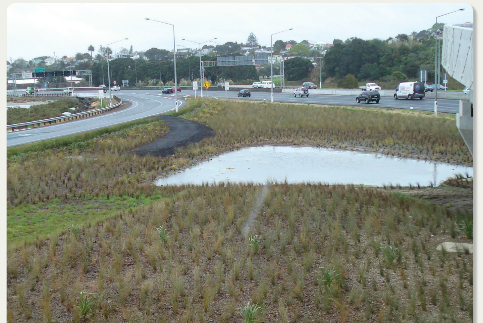
Example of stormwater treatment basin
