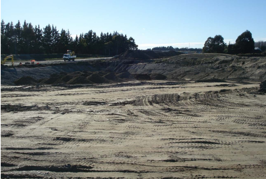
Figure 9 Excavations at the Owaka Pond Site
