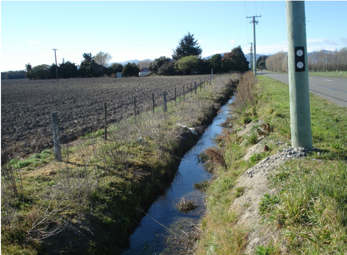
Figure 6 Existing Stockwater Race along Marshs Road
