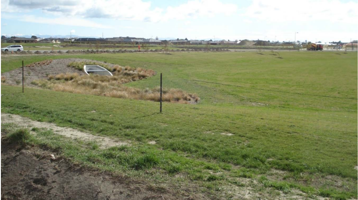
Figure 10 Example of Engineered Stormwater Detention Basin Adjacent to Awatea Road
