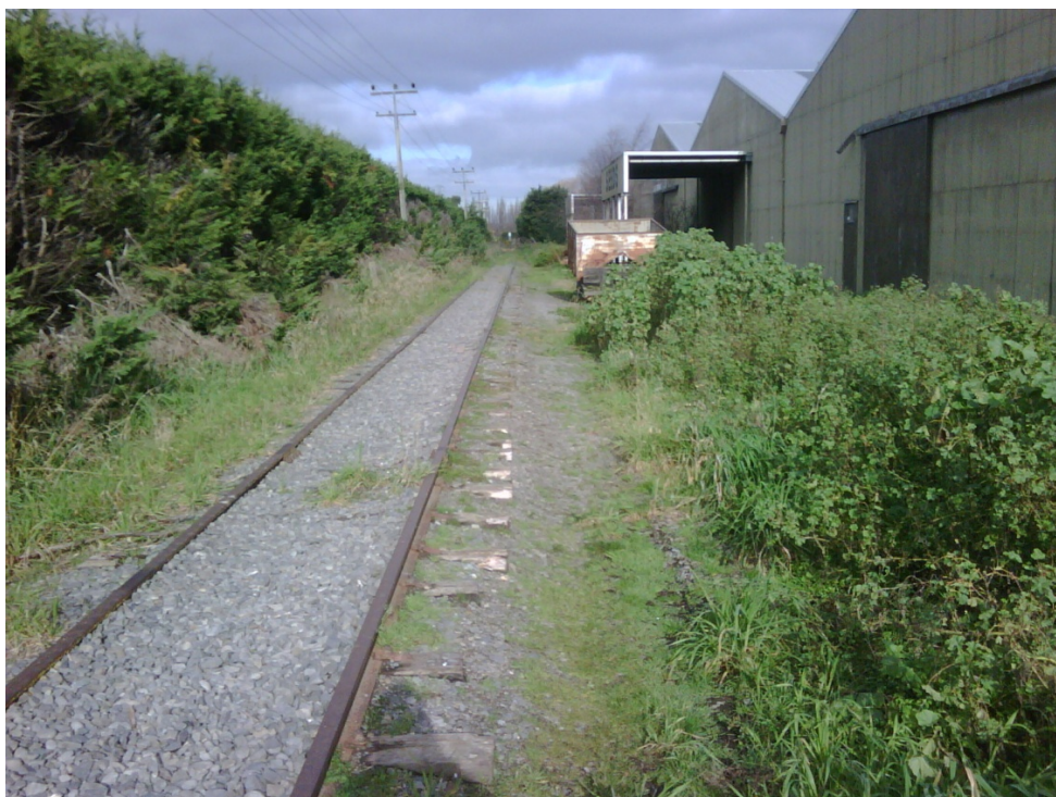
Figure 8 Photograph of former Southbridge Branch Railway Line looking South (1 July 2011)
