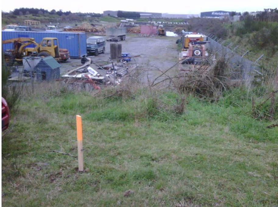
Figure 2 Photograph of Compound Area Looking West (30 June 2011)
