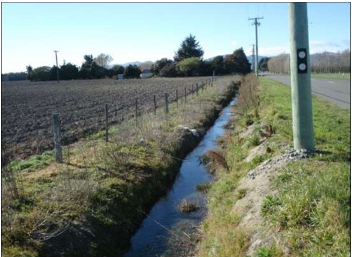
Figure 9: Marshs Road water race
