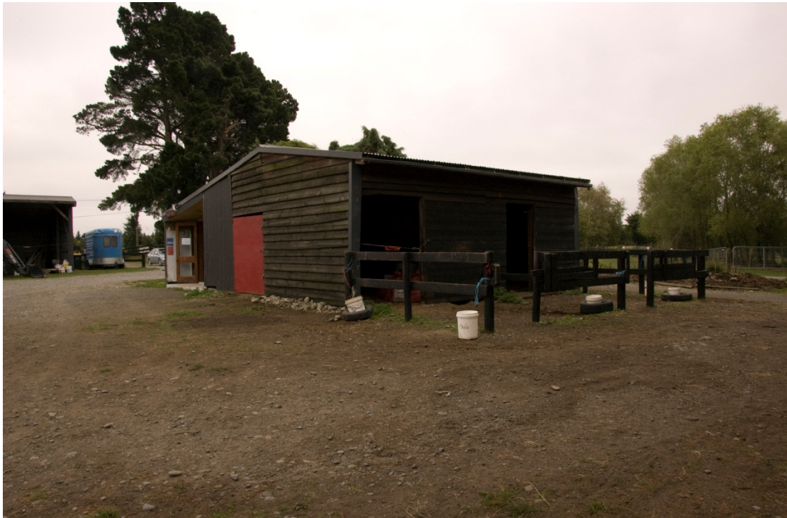
Figure 7. The shed, 2 April 2012.
