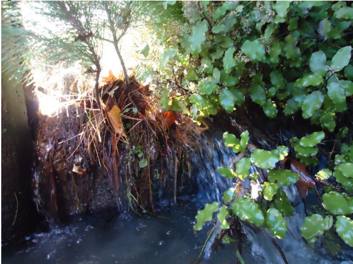
Figure 3 Weir at the intersection of Trents Road and Blakes Road
