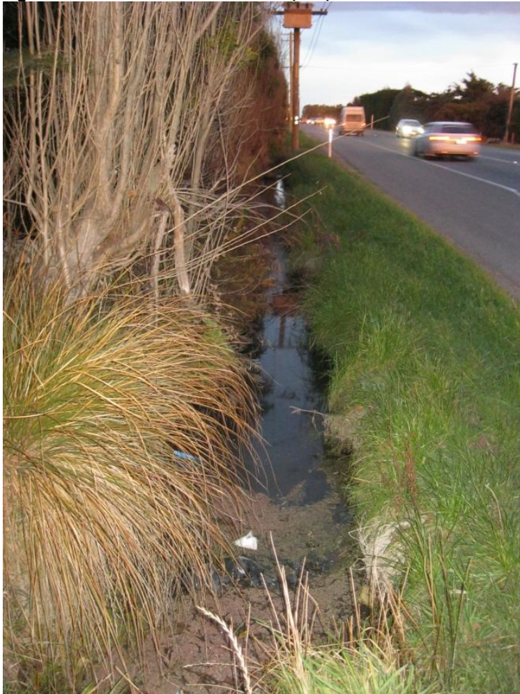
Figure 1 Site A – Main South Road (SH1) near Berketts Road
