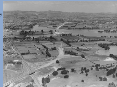
Takanini Interchange under construction - looking south, 19 November 1963 (Credit Alexander Turnbull Library Ref:WA-61078-G)
