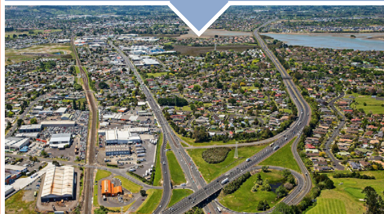
Takanini Interchange 11 November 2015, just prior to the start of works
