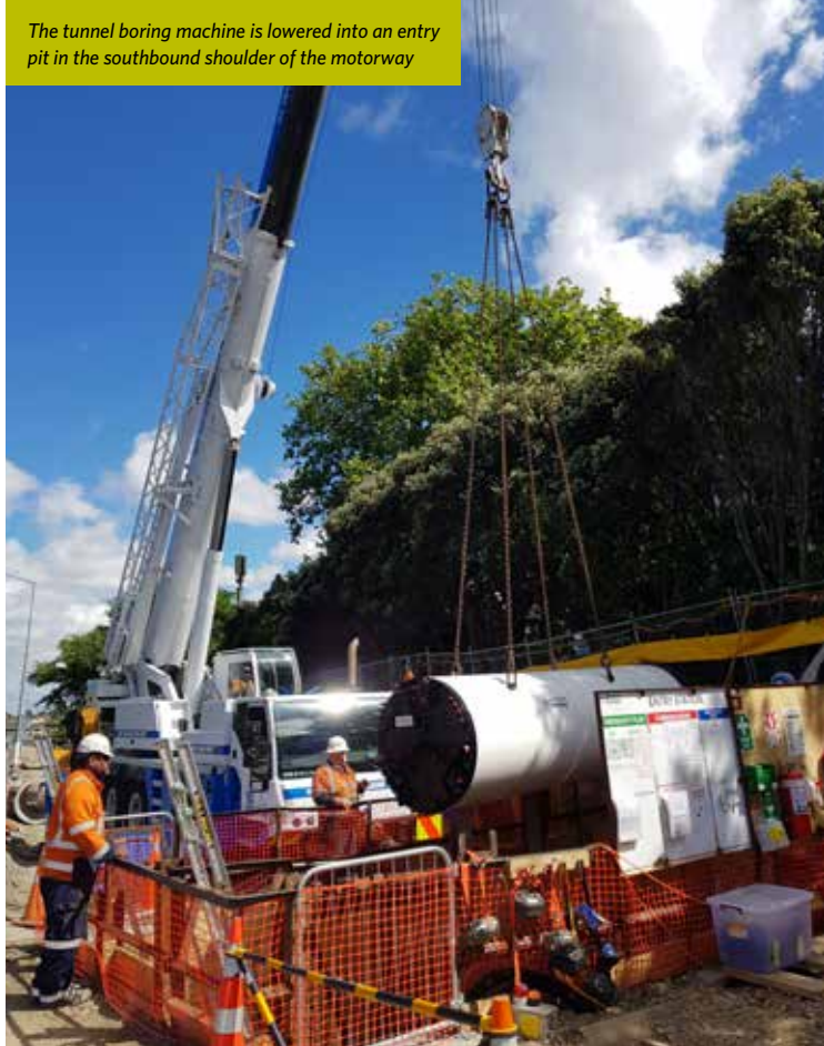
This tunnel boring entry pit near Auckland Botanic Gardens is 4.5 metres deep and the machine itself will bore underneath the motorway
