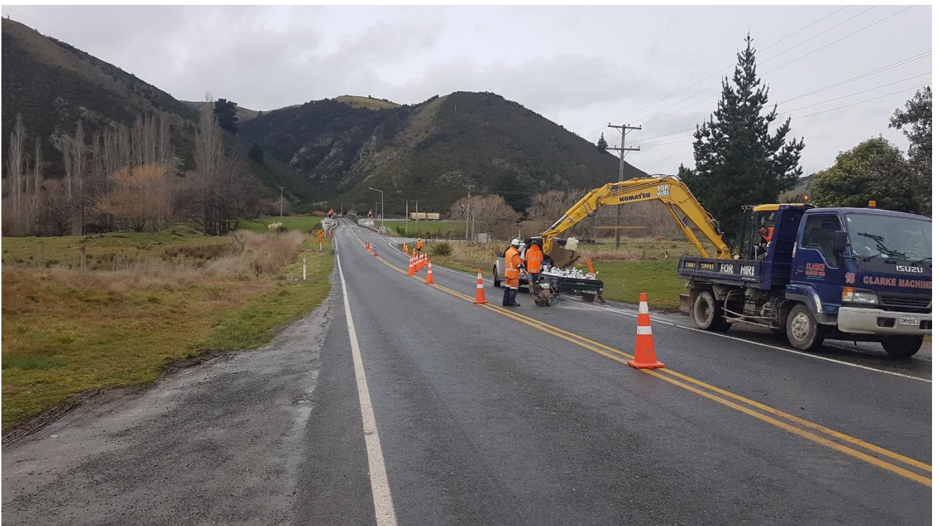
Photo 10: SH8 western side towards existing bridge
