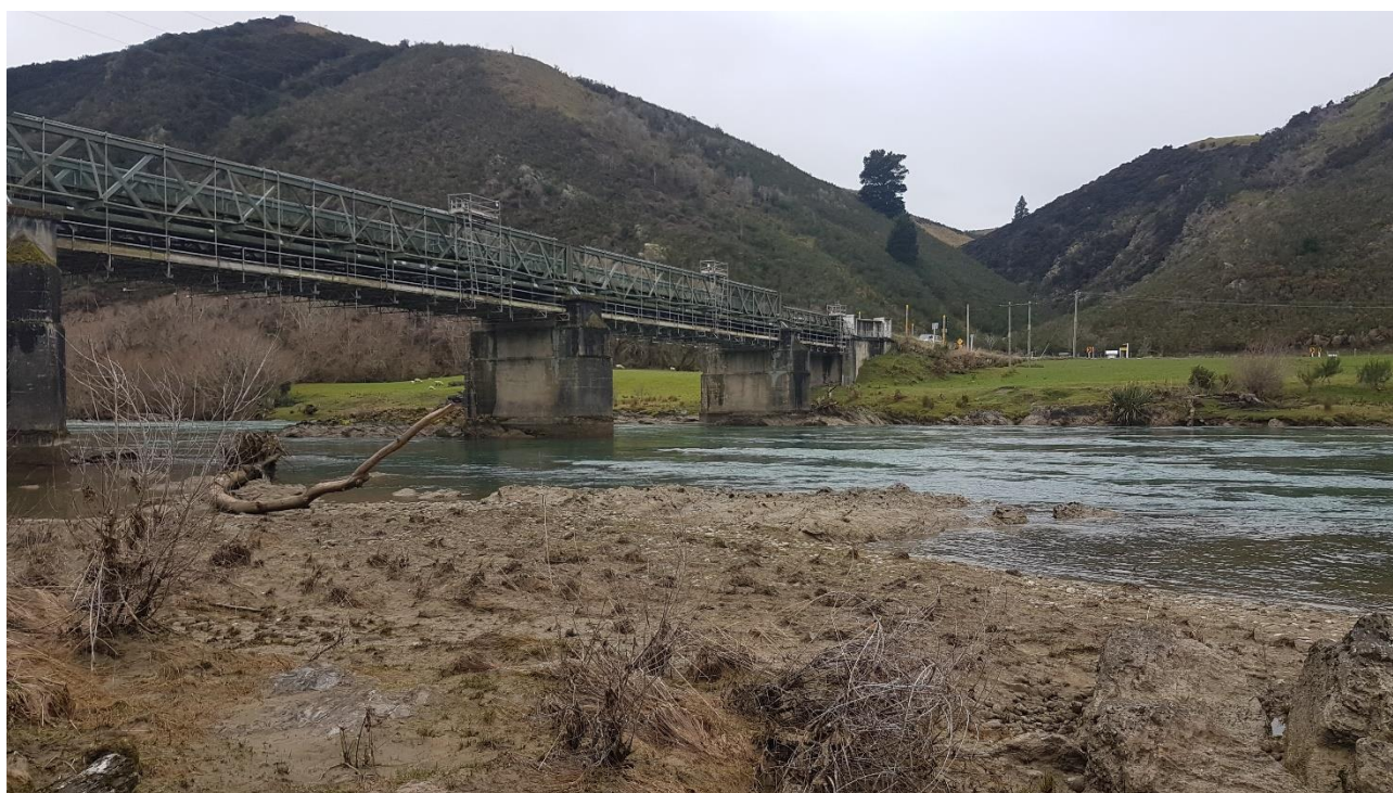
Photo 6: Eastern bank and existing bridge viewed from western bank
