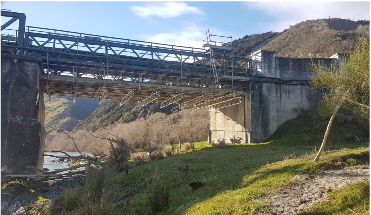
Photo 4: Eastern abutment of existing bridge
