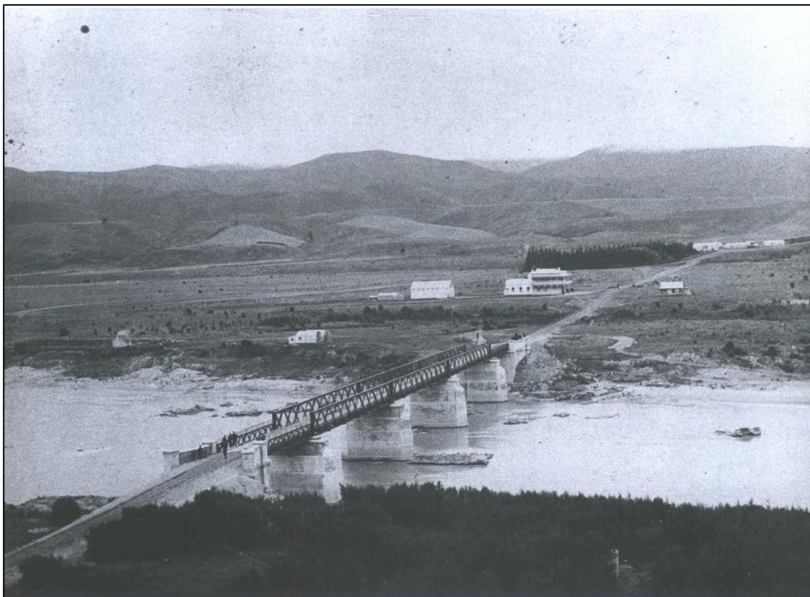
Figure 12. Photograph looking at the second and current Beaumont Bridge c.1890 (source: Hocken Collection Asset ID 6264)
