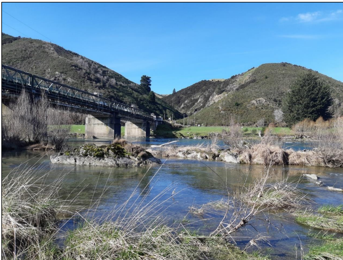
Figure 21. Photograph looking east of the Beaumont Bridge in the background and the Project area in the foreground
