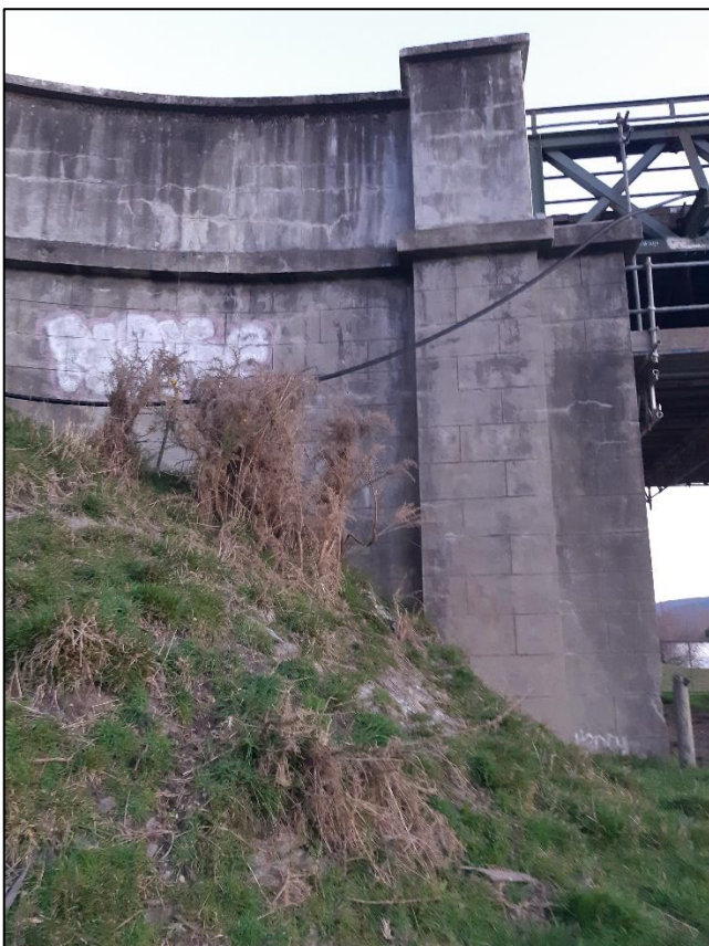
Figure 22. View looking south of the eastern Beaumont Bridge abutment, showing the built-up bridge approach in foreground
