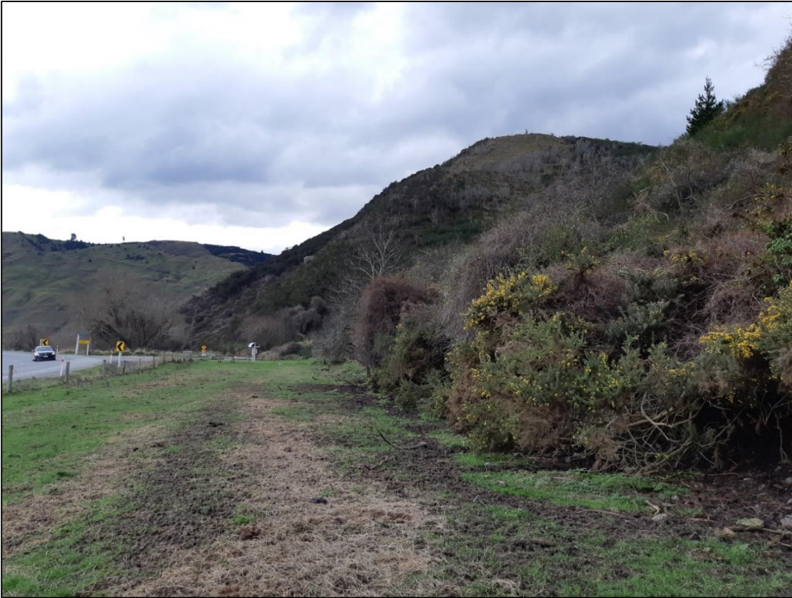
Figure 17. Photograph showing the old rail alignment looking north from further west
