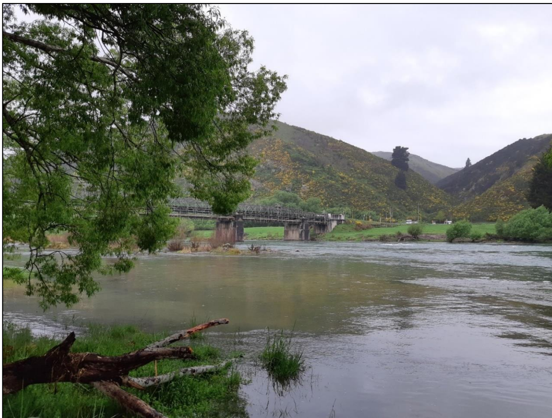
Figure 23. View of the Beaumont Bridge from downstream on the true right
