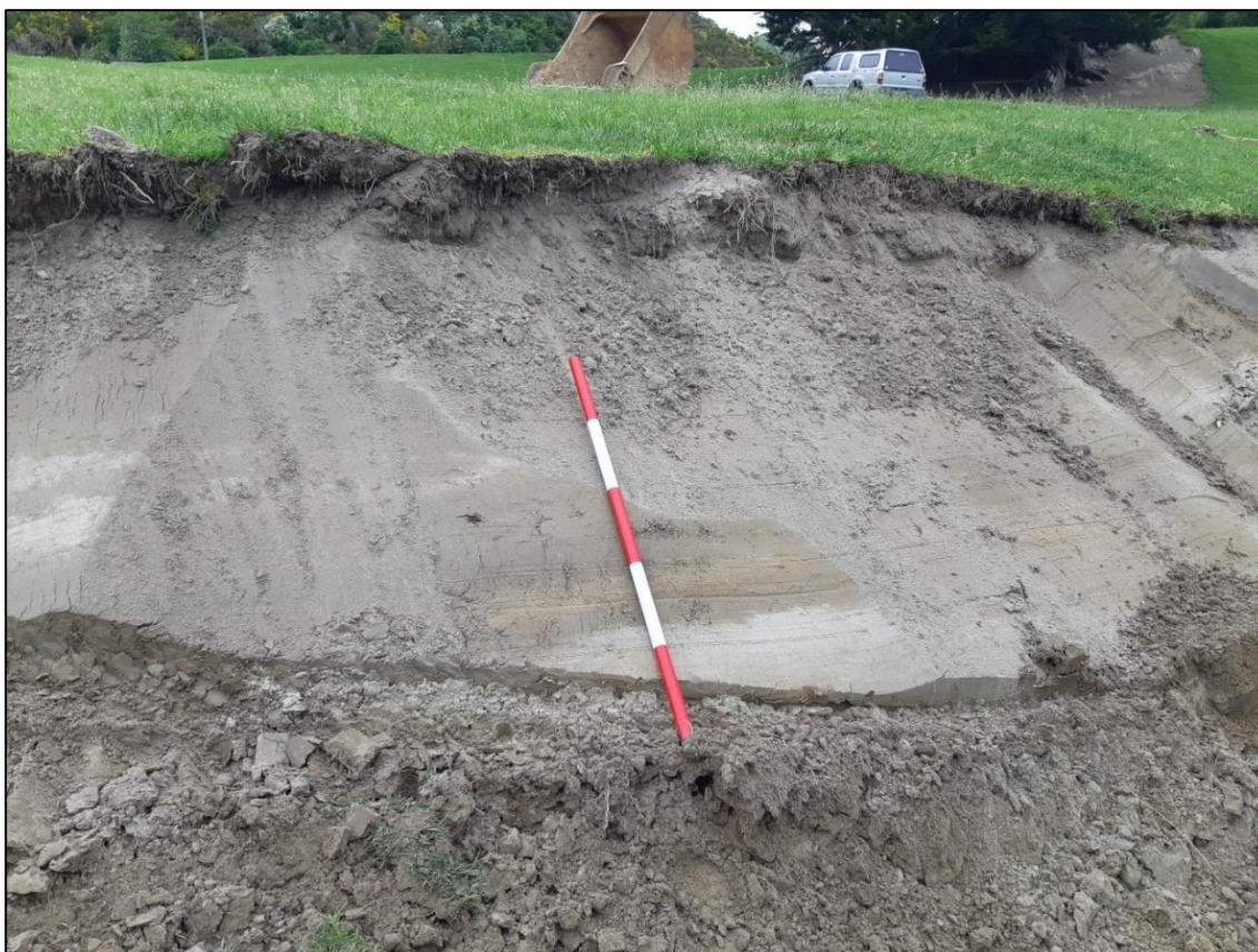
Figure 20. Photograph detailing a batter edge on the true left of the bank of the Mata-au
