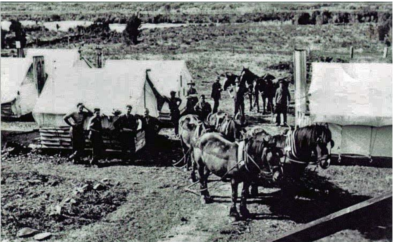
Figure 17: Forestry Camp at Tramway near Beaumont, 1920s.
