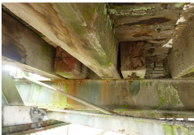
Figure 37: Timber bearers on wrought iron transom.
