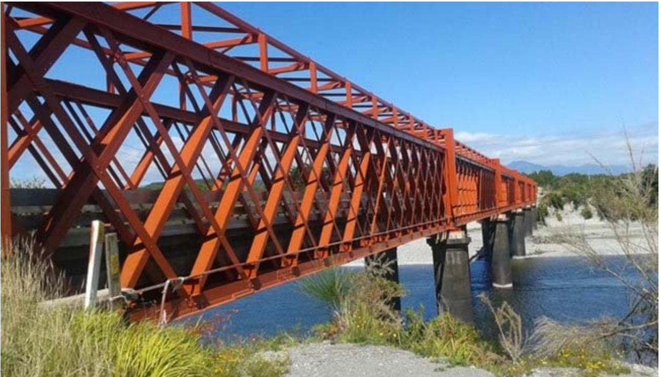
Figure 44: Taramakau Road and Rail Bridge, SH6.
