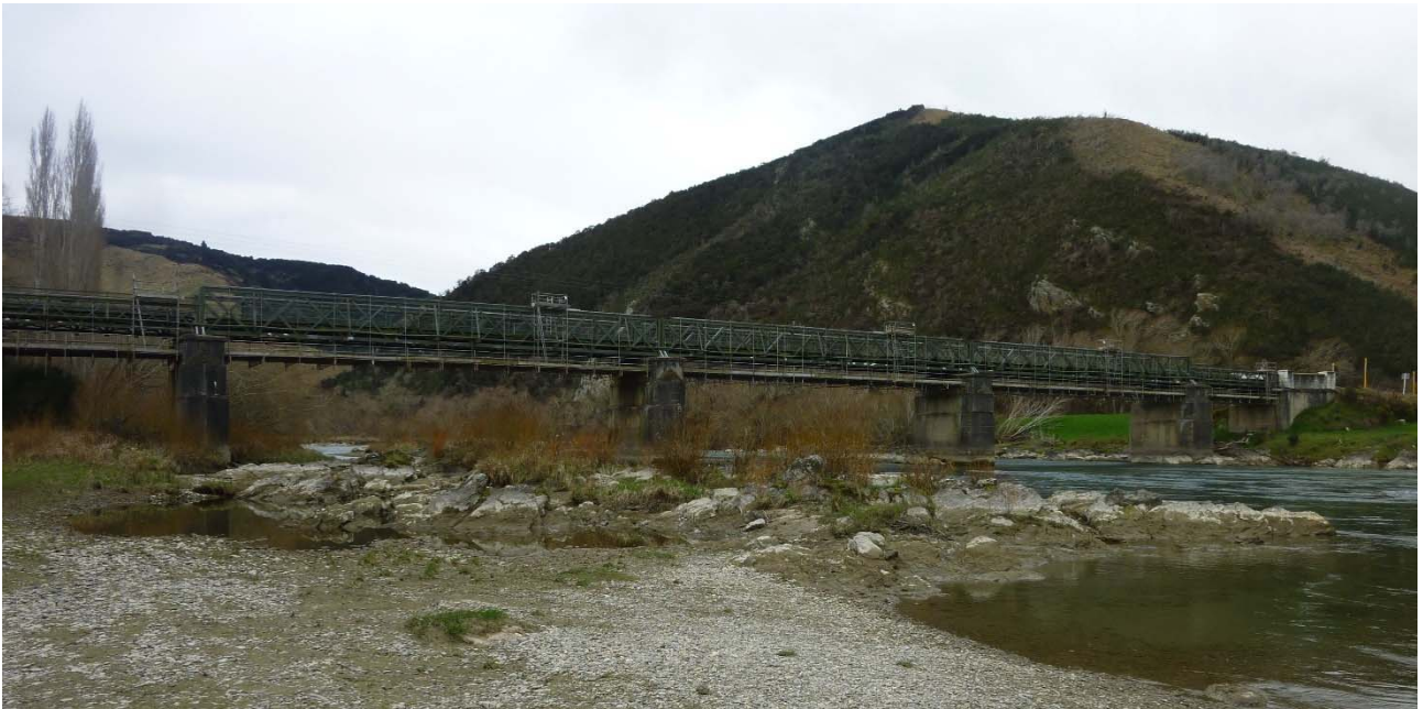
Figure 28: Beaumont Bridge viewed from south.
