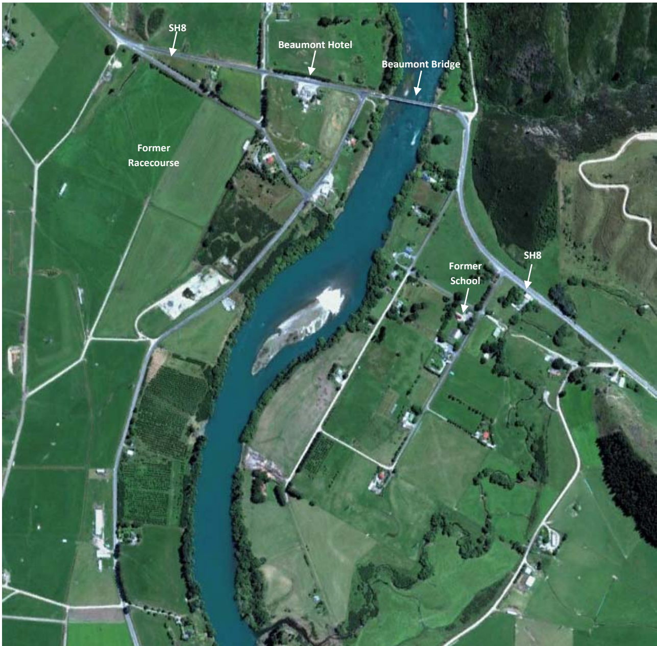
Figure 3: Aerial photo showing location of Beaumont Bridge in relation to the Beaumont Township.
