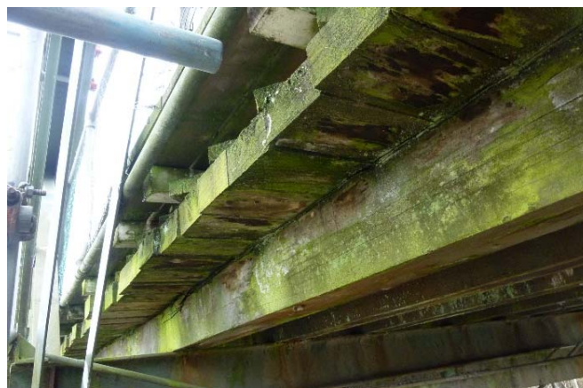
Figure 38: Timber bearers and edge of timber decking.
