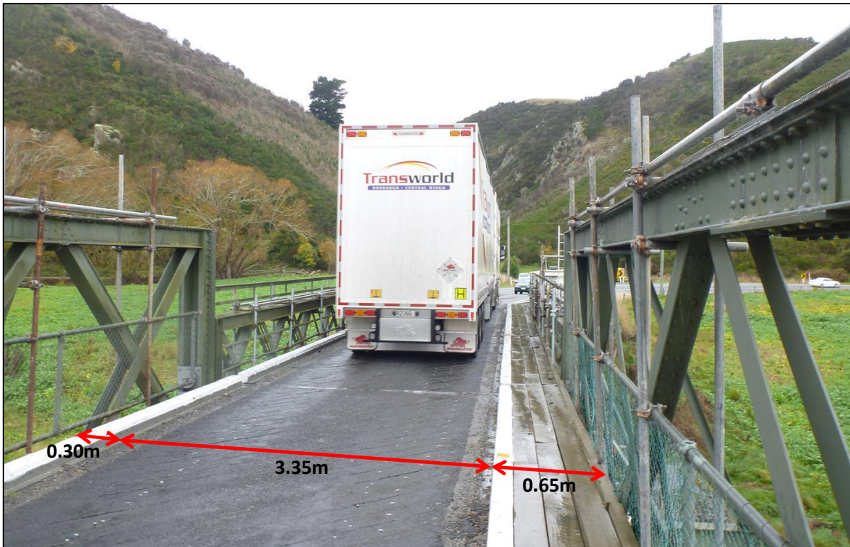
Figure 3: Existing Bridge Configuration
