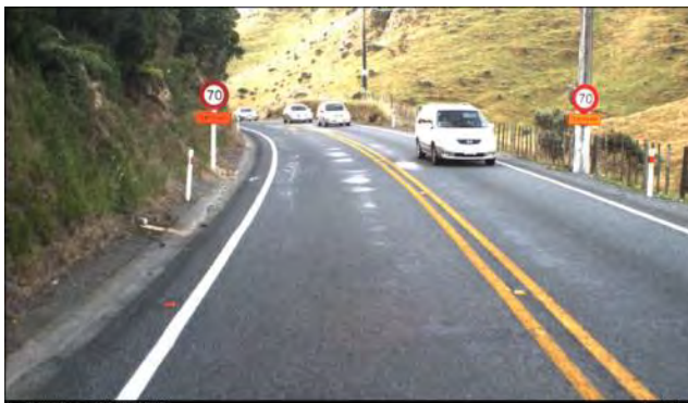
Figure 3-5: Approach to the existing 70 km/h 'temporary' signage and first curve in the 'broken back' alignment heading west (Increasing)
