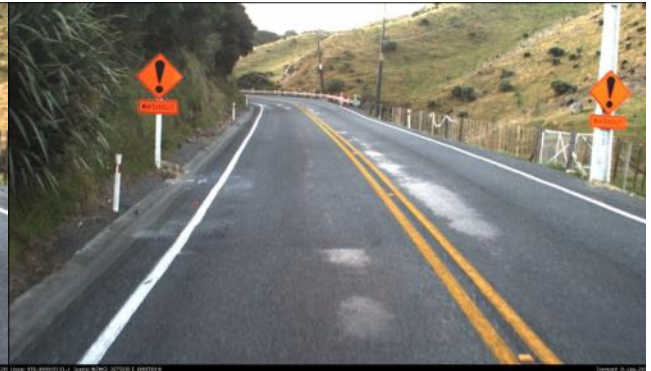
Figure 3-7: Second curve in the 'broken back' alignment heading west (Increasing)
