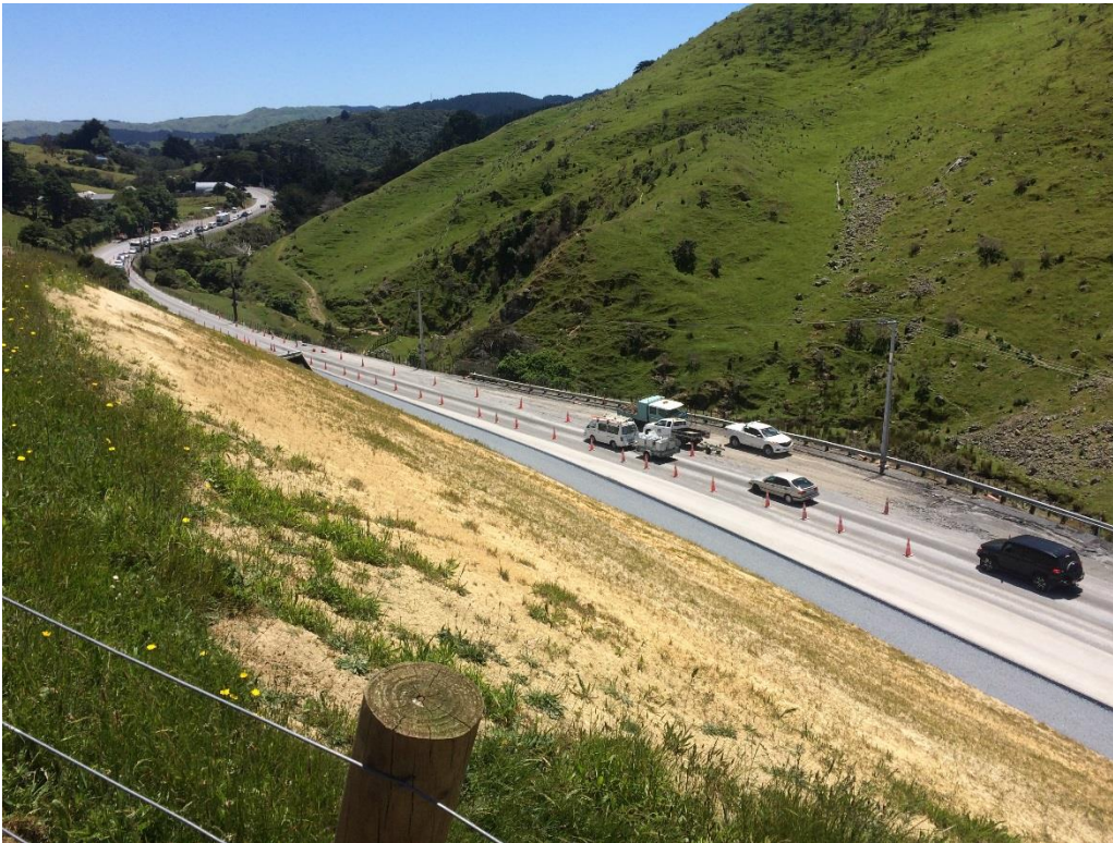
Figure 6-3: Photograph of Scour Site Realignment works during construction
