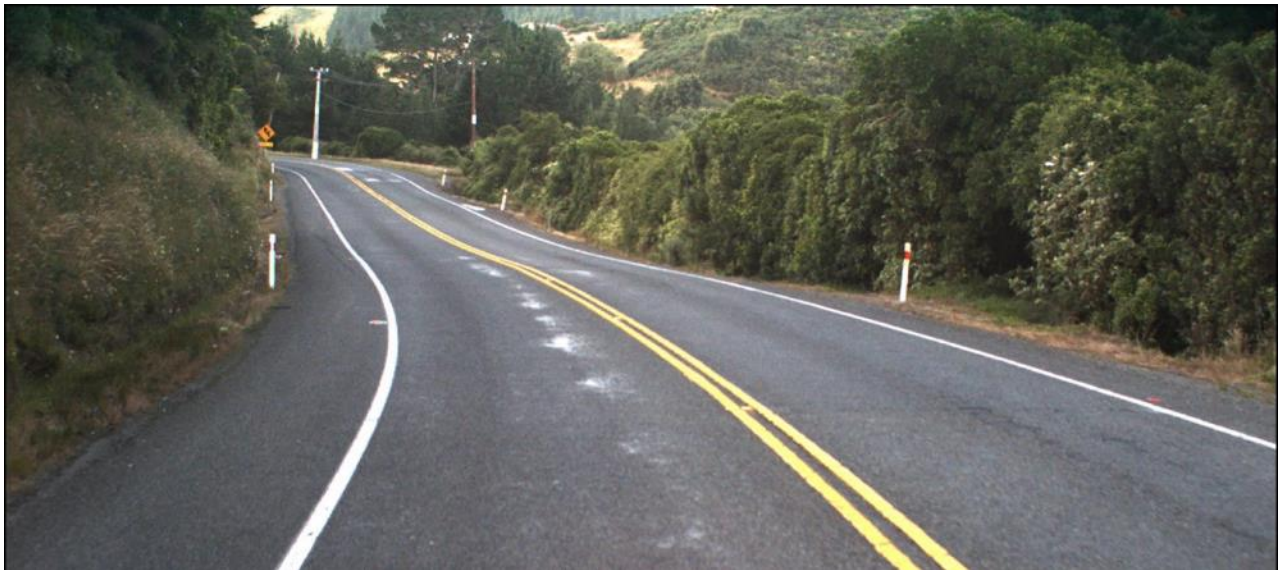
Figure 3-5: Approach to the short straight between the two left hand curves in the 'broken back' alignment heading west (Increasing RP 0/2.58)
