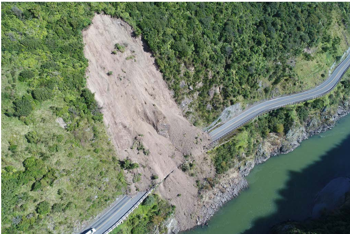
Figure 1-3 Photograph of Anzac Slip, April 2017
