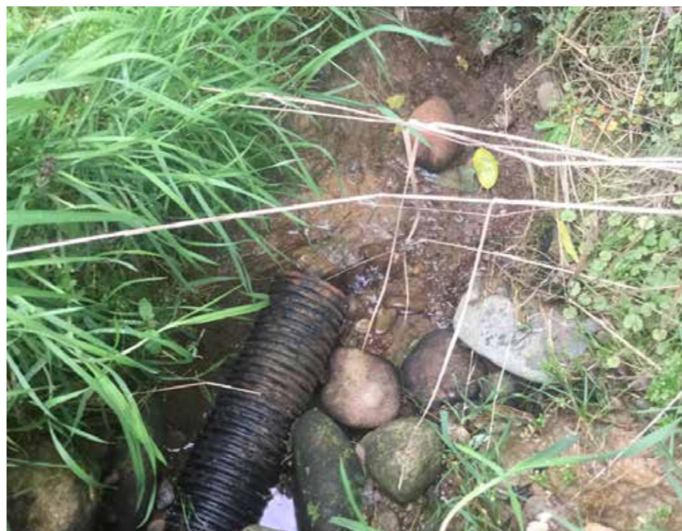
Stream 6A1 downstream end of novocoil pipe under farm track at top of Catchment 6A
