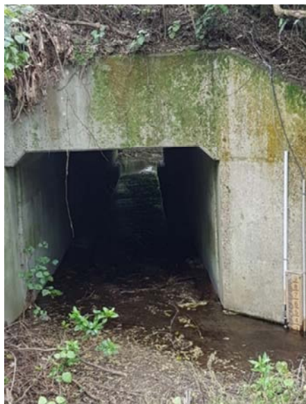
Figure D.24: Water level and turbidity sensors at the upstream end of the culvert under the railway embankment on Stream 7.
