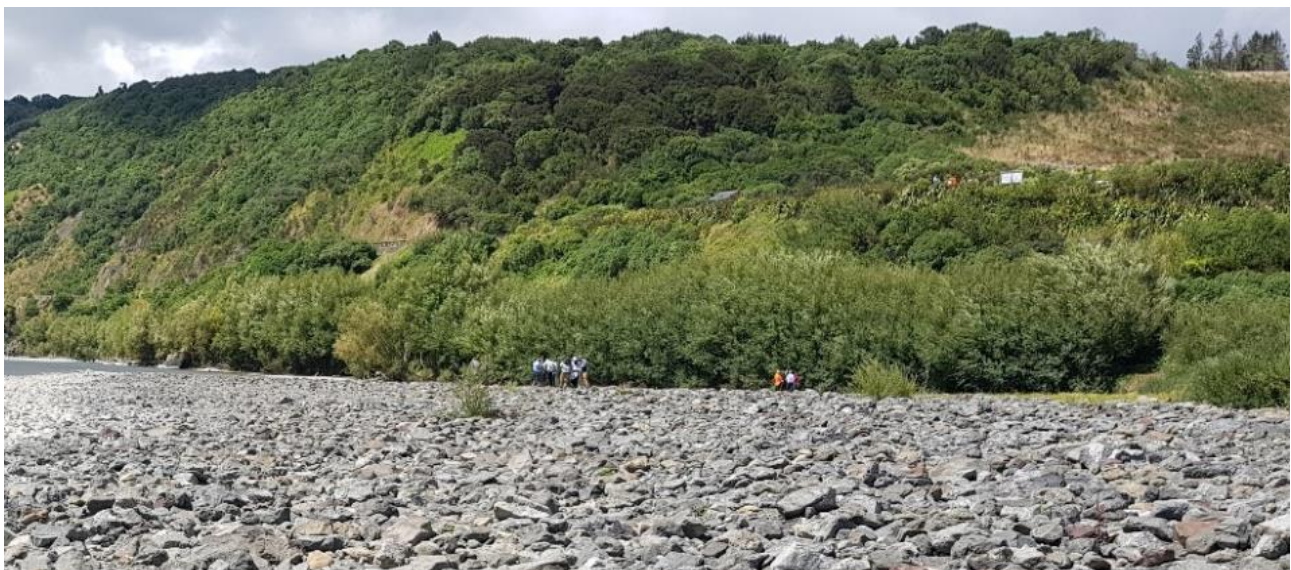
Figure 5-1 Manawatū River channel looking upstream from Parahaki Island with existing vegetation near proposed Pier 1 on the true right bank.
