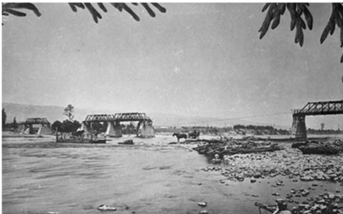
Figure D.7: The collapse of the Ashhurst Bridge in 1885.
