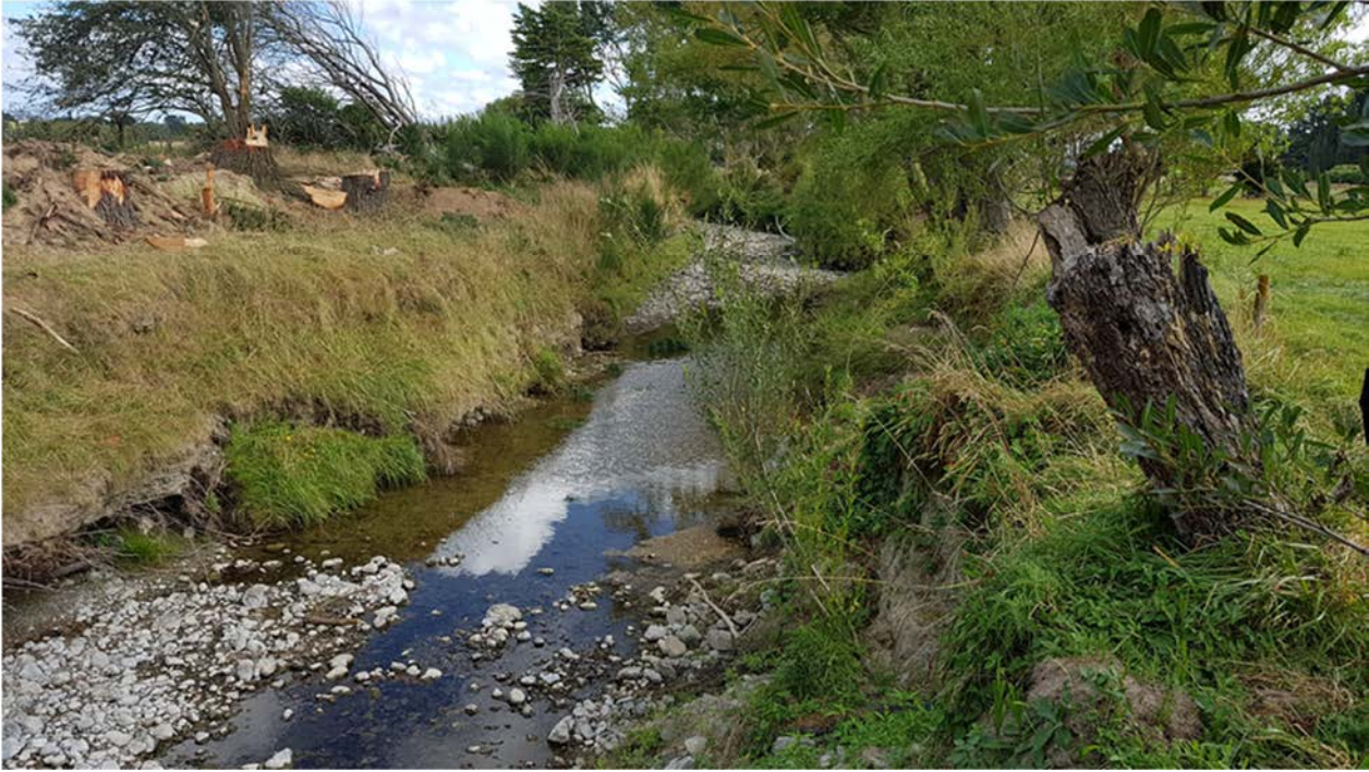
Figure 3-2: Mangamanaia Stream Bed
