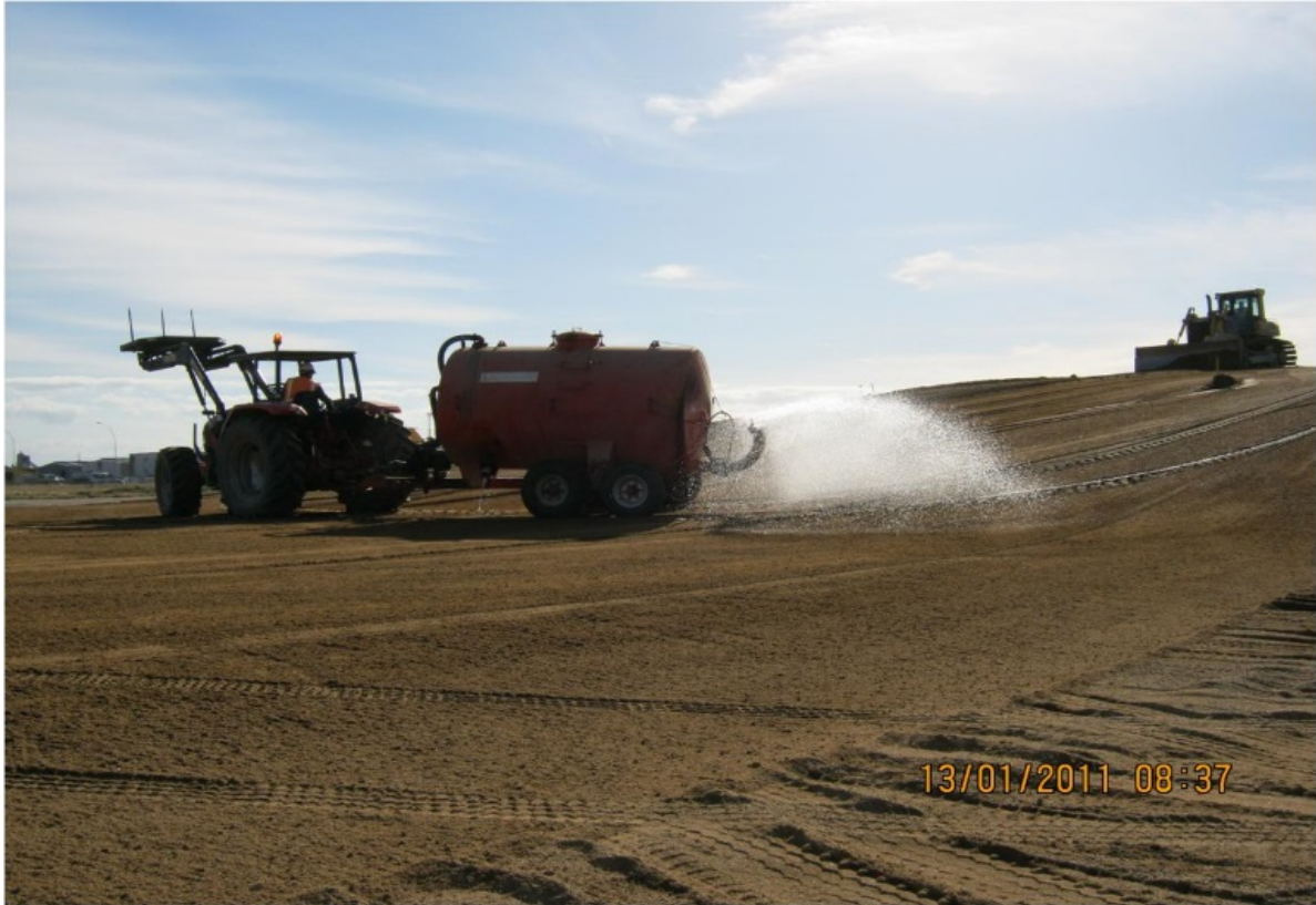
Photo 2: Water Tanker in Operation
