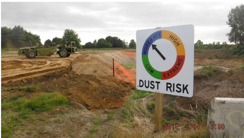
Photo 3: Dust Risk Signs will assist with Communicating the Risk to Construction Staff
