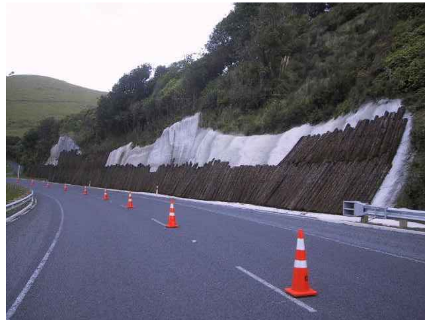
FIGURE 1 - PONGA LOGS FIXED OVER THE SHOTCRETE (SH3 MOKAU) N.T.S.
