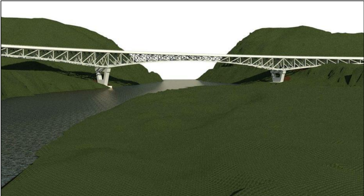
Figure 5: Artist concept of Manawatū River Bridge 2 Option A: No Piers in River (from NOR documentation lodged in November 2018)
