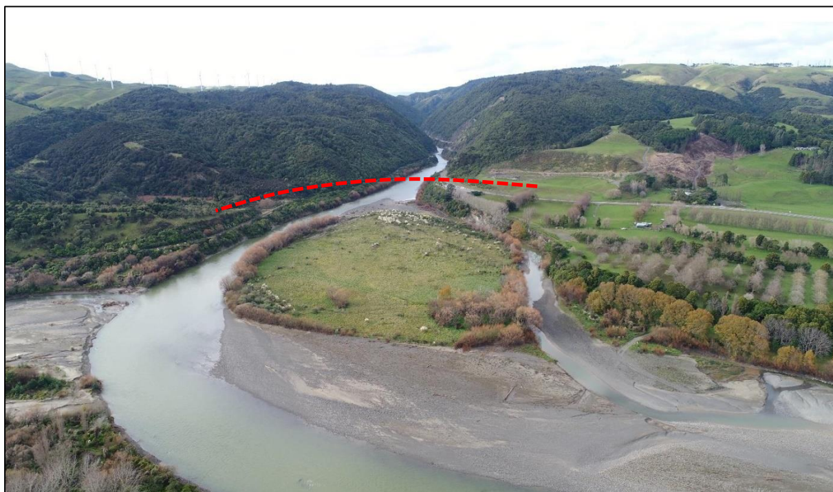
Figure 12: View east at mouth of Manawatū Gorge over Parahaki Island with proposed new bridge indicated by red dotted line (adapted from NZTA)
