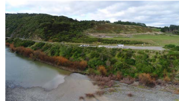
Figure 14: Car park and location of the proposed south bridge abutment.
