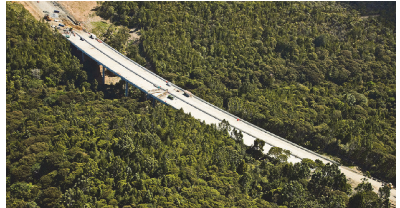
Figure 8: Otanerua Eco Viaduct under construction. Northern Toll Road
