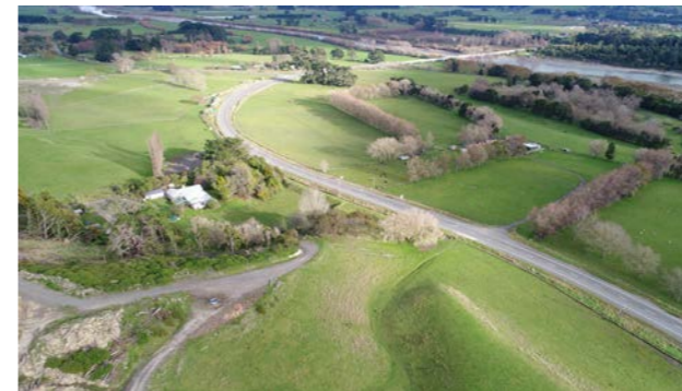
Figure 16: View west with the existing SH3 bridge in distance.
