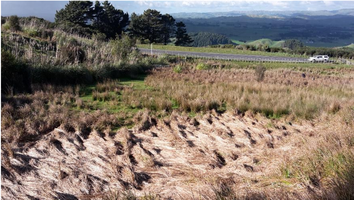
Figure 6.B.33. The wetland area between approximately Ch 10200 and Ch 10280 by Saddle Road.
