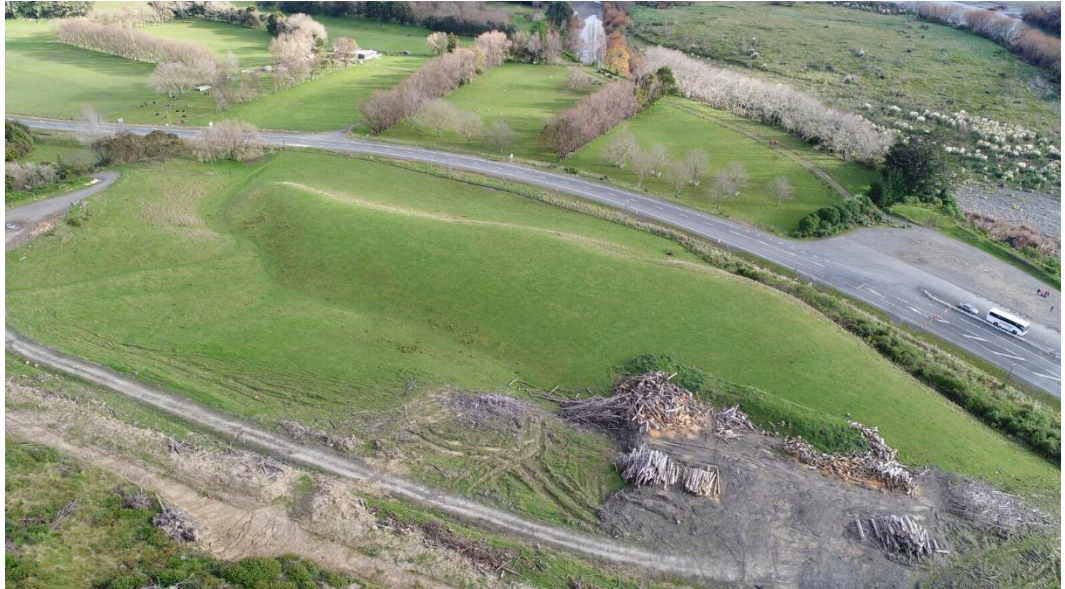
Figure 24. The plateau to the south of the existing SH3 and Manawatū River
