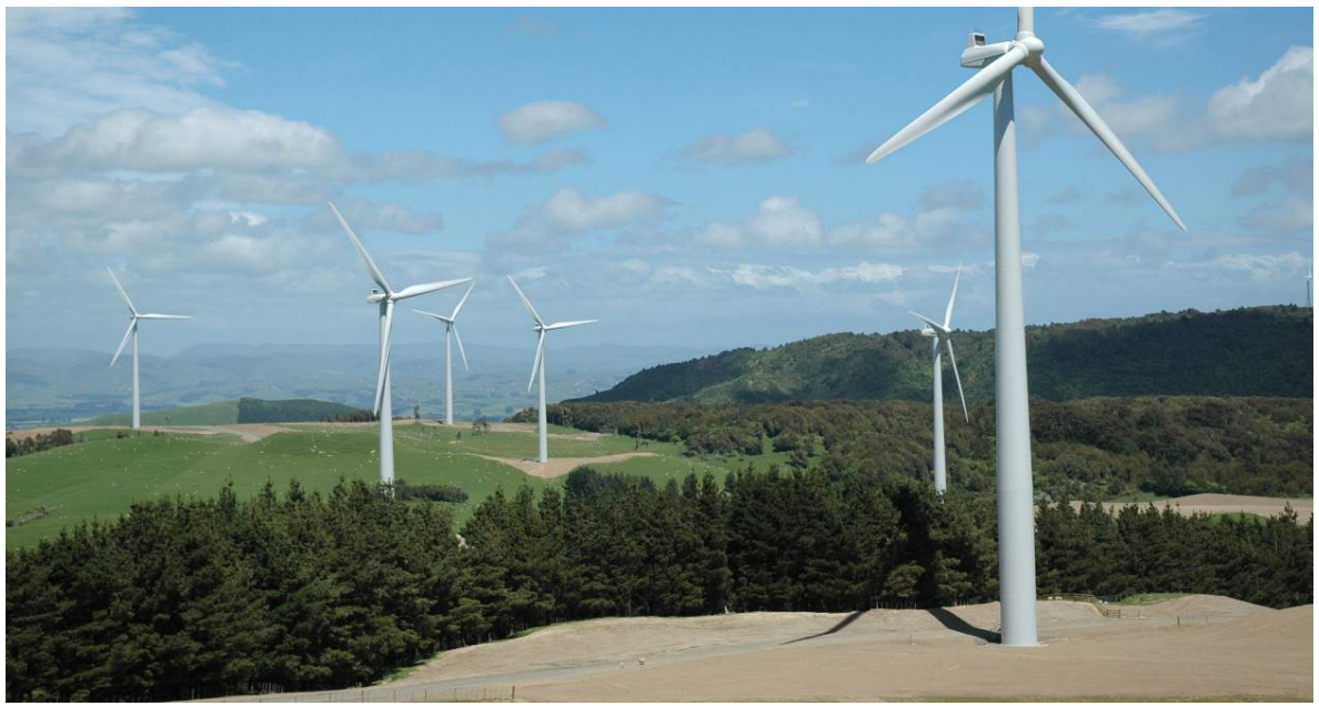
Te Apiti Windfarm, Palmerston Nth, North Island
