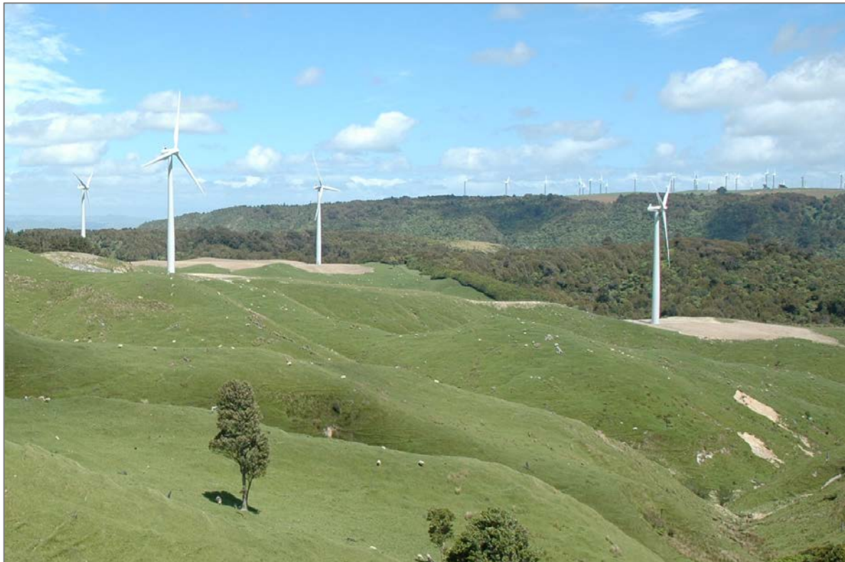
Figure 4: Typical 1.65 MW wind turbines at Te Apiti wind farm (70 m high supporting column with 35 m blades). Also note the edge of Manawatu Scenic Reserve behind the turbines.
