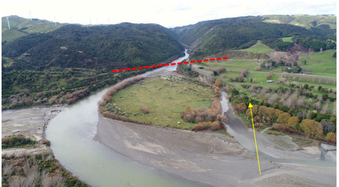
Figure 25. Looking east into the Gorge at the confluence of the Manawatū and Pohangina Rivers. Moutere Island (Parahaki) is in the middle ground. The new Project bridge will cross the Manawatū River and Palmerston North to Gisborne Railway line at the mouth of the Manawatū Gorge, to the south of Moutere Island and to the north of the Manawatū Gorge Scenic Reserve (dashed line). Location of karaka trees (T24/31) arrowed.
