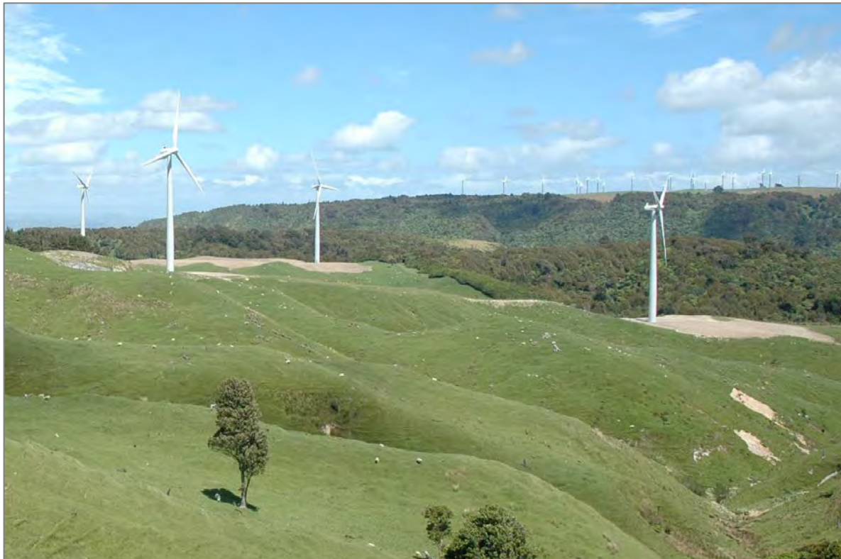
Figure 4: Typical 1.65 MW wind turbines at Te Apiti wind farm (70 m high supporting column with 35 m blades). Also note the edge of Manawatu Scenic Reserve behind the turbines.
