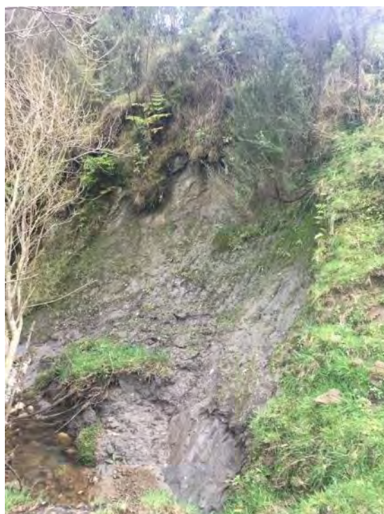
Image 6.C.26: Bank slumping along the western main stem (5B).
