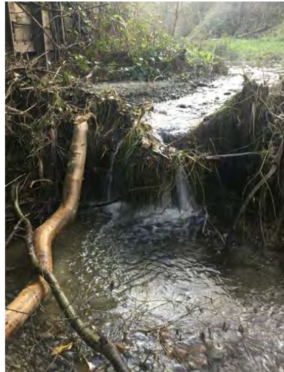
Image 6.C.34: Downstream reach of the main stem (7A). Note the stream flowing over a retaining wall structure reducing fish passage.
