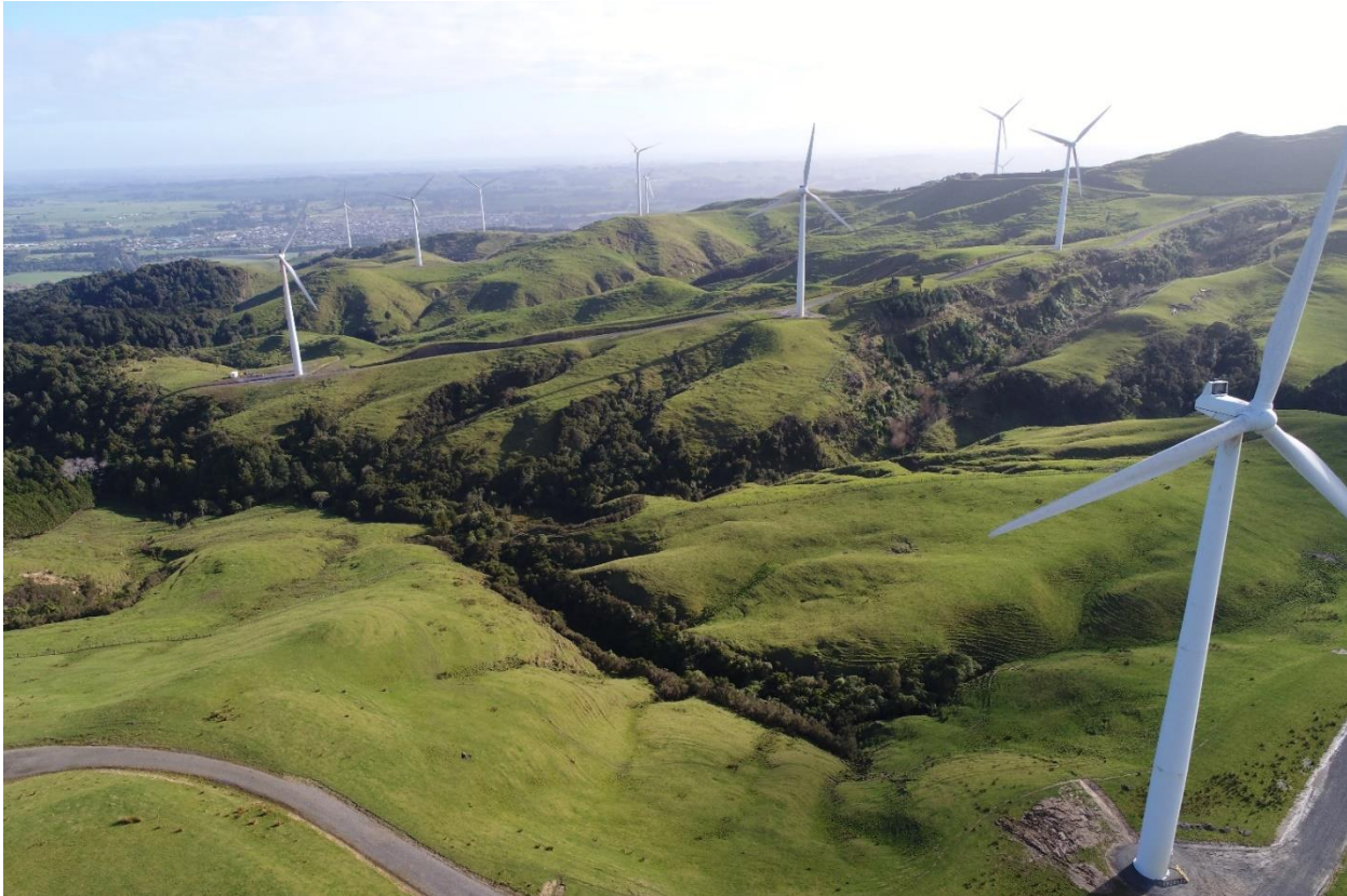
Figure 8 – View west across Te Āpiti wind farm towards Ashhurst
