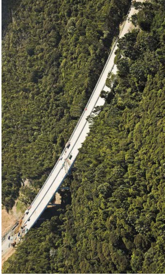
Figure 8: Otanerua Eco Viaduct under construction. Northern Toll Road
