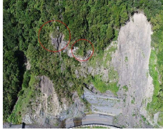
Figure 6 Aerial view of Kerry's Wall slip site (cracks circled in red)
