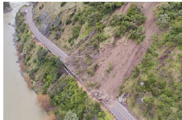
Figure 8 Aerial view of slip that occurred in the Manawatu Gorge on 23 July 2017
