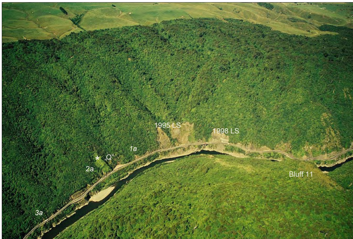
Figure 11. January 2000 photo of the 1995-1998 landslide works and „Quarry” in the Manawatu Gorge showing the areas (1a, 2a, 3a) where landslides #1, #2, and #3 occurred in February 2004. A shallow debris slide occurred at the landslide #2 site during the 1960s (note the young vegetation*).
