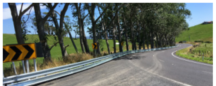
Barrier with motorcyclists protection system (example)
