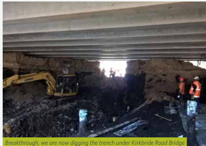
Breakthrough, we are now digging the trench under Kirkbride Road Bridge
