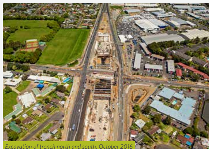
Excavation of trench north and south, October 2016
