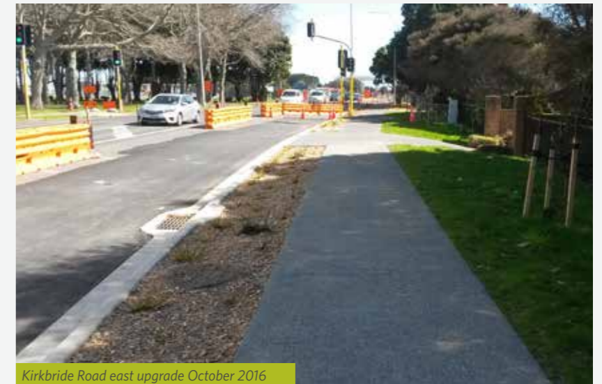
Kirkbride Road east upgrade October 2016
