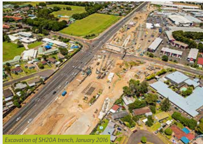
Excavation of SH20A trench, January 2016
