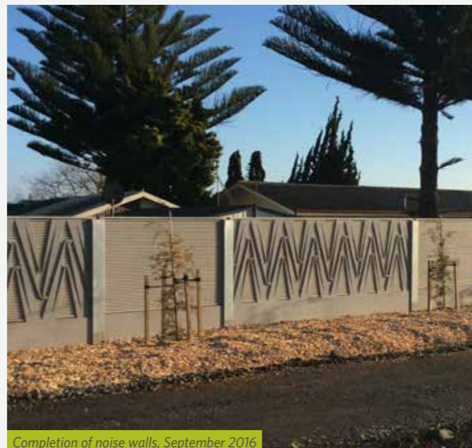
Completion of noise walls, September 2016
