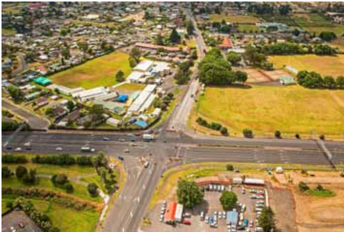
The Kikbride Road/ SH20A intersection in January 2015 .
