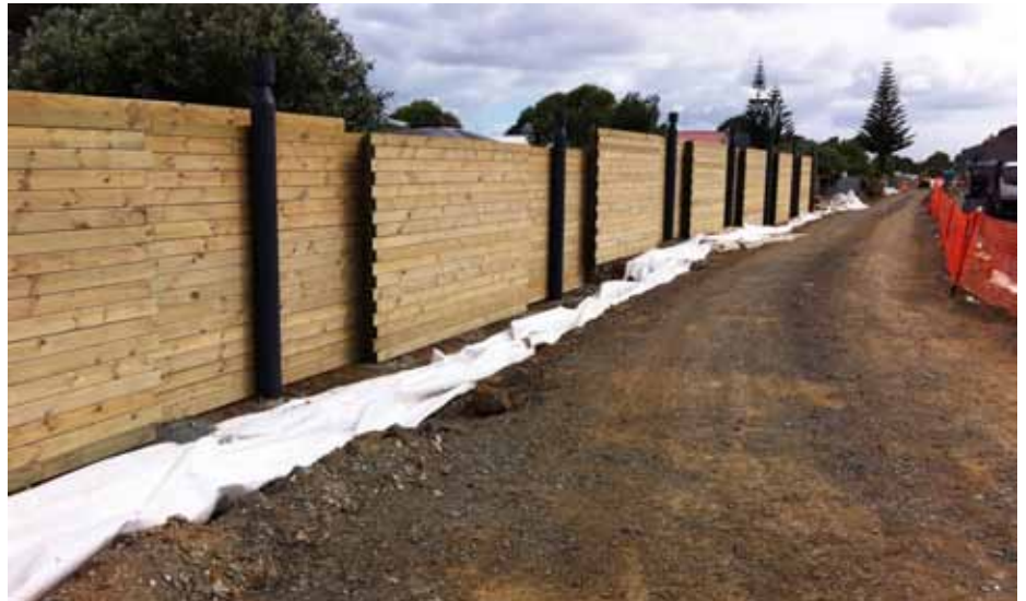
The timber noise walls incorporate 'pou-like' poles and appear to step in and out giving depth to the surface
