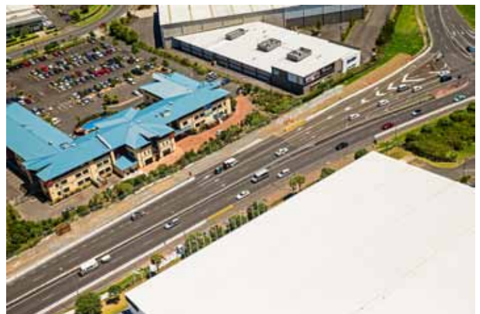
Beginnings of the shared pedestrian and cycle path near the Montgomerie Road/ SH20A intersection.
