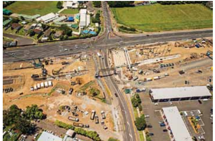
The Kikbride Road/ SH20A intersection in January 2016 .
