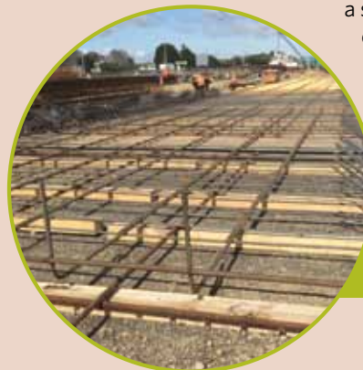
Cages being prepared to use for construction of the d-walls.
