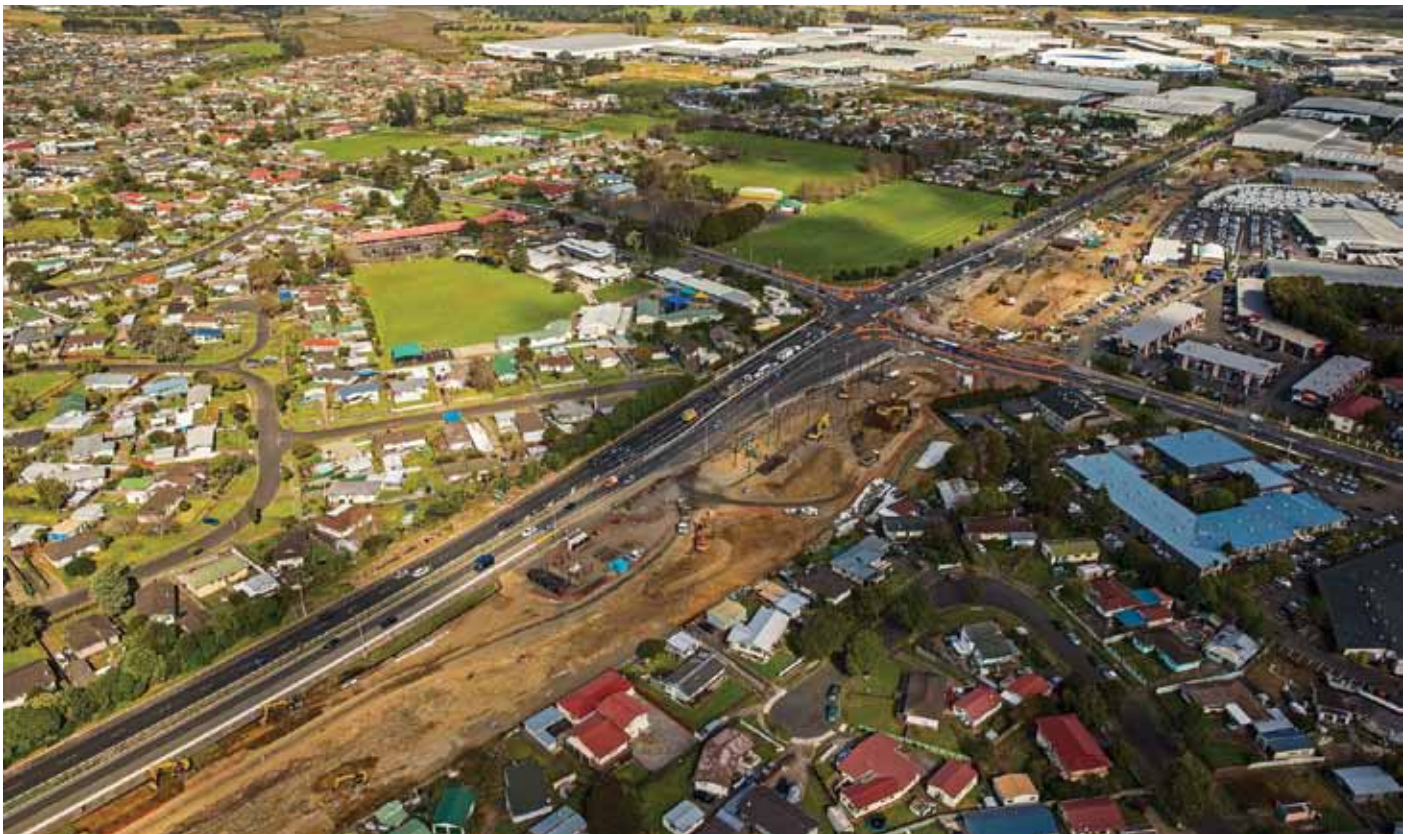
Construction progress, August 2015.
