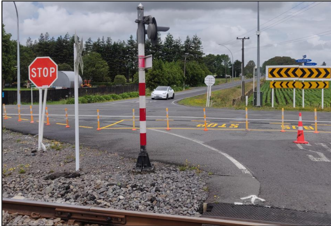
Figure 3-5: Bus Stop within the intersection
