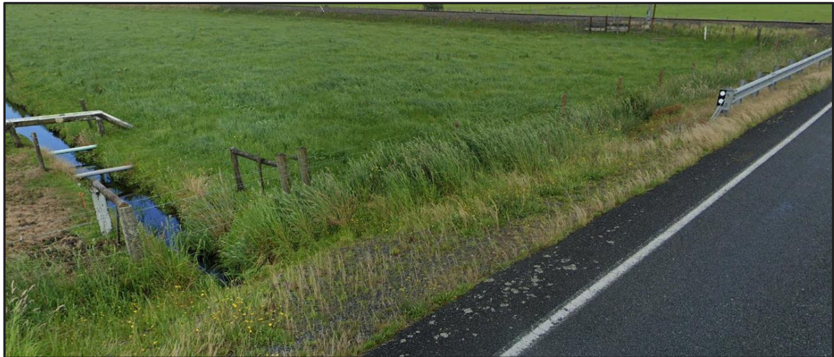
Figure 4-8: Waverley Drain Crossing
