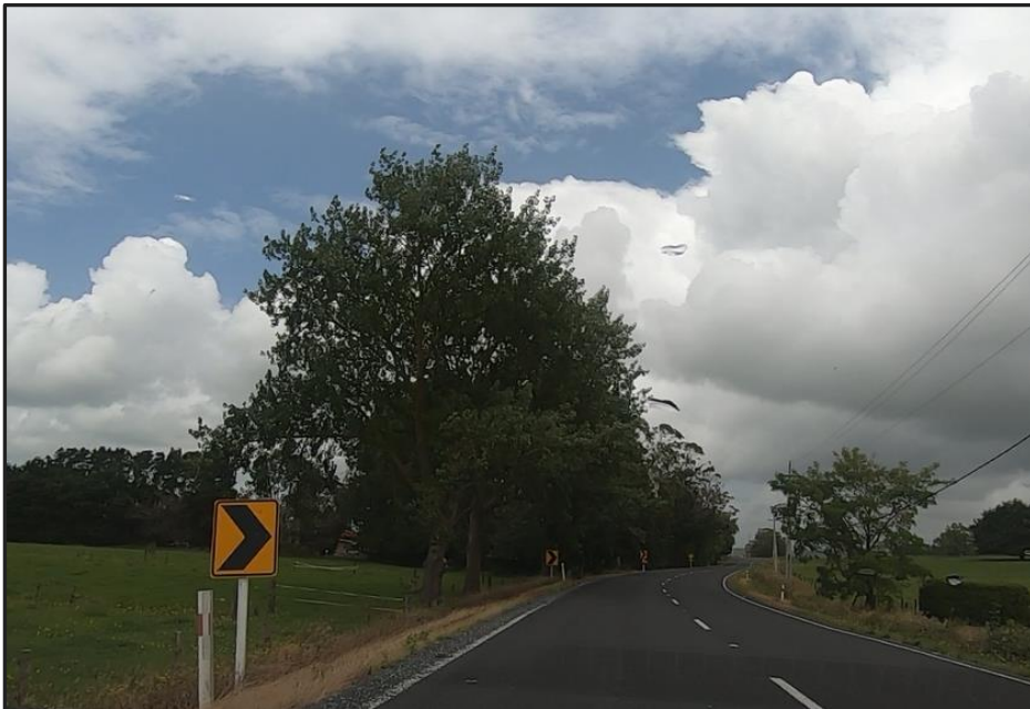
Figure 4-3: Road side drop off at CH4560 with large non-frangible trees
