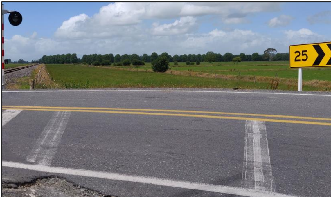
Figure 4-10: Steep drop off behind the 25km/h sign
