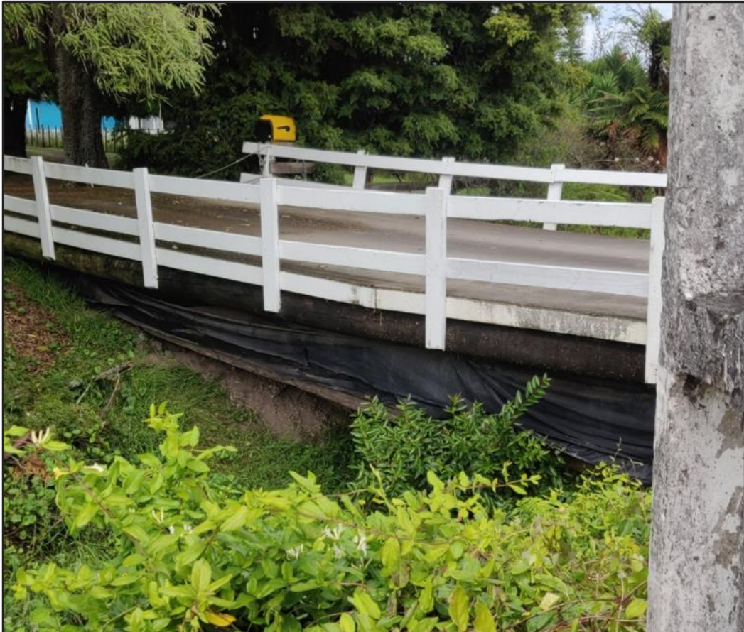
Figure 3-4: Deep side drains and driveway crossing on Telephone Road
