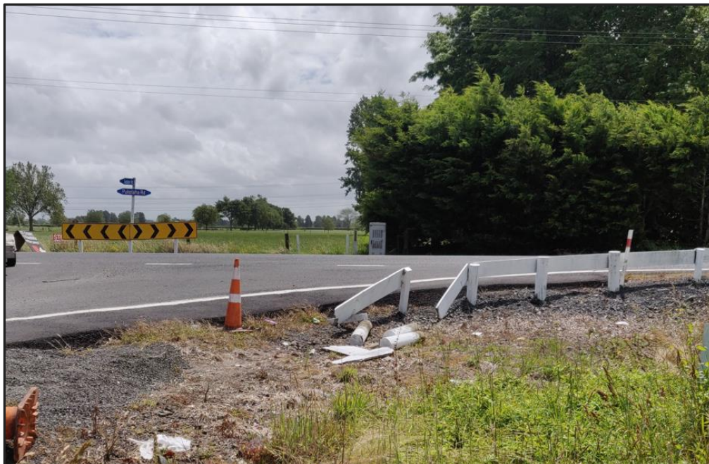
Figure 4-2: White sight rail on the northern side
