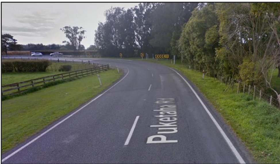
Figure 3-1: Puketaha Road (2017) no signage installed
