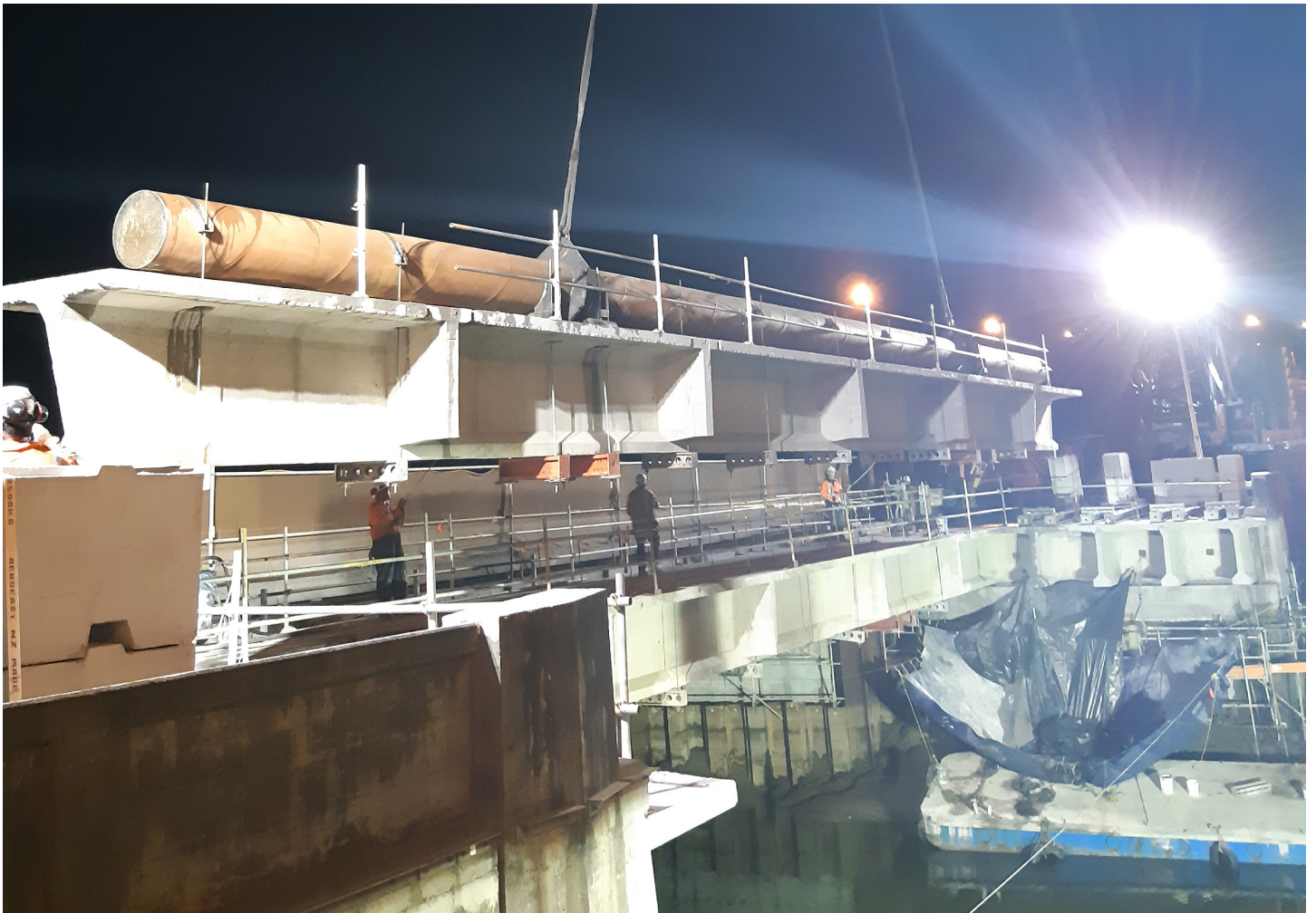
Removal of the bridge deck of the old bridge structure.
