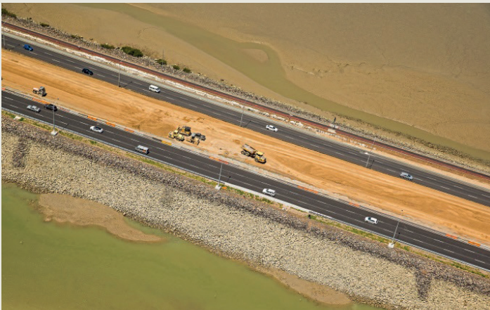
The team is now working in the median areas along the causeway, building up the existing motorway ready for its final surface and traffic later this year.
