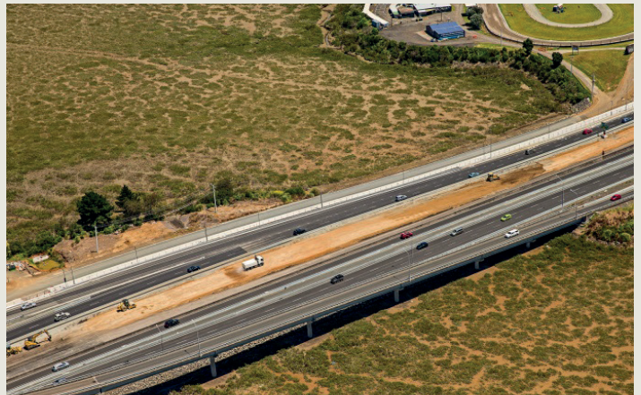
The team is now working in the median areas along the causeway, building up the existing motorway ready for its final surface and traffic later this year.
