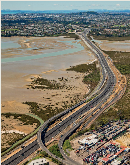
Earthworks either side of the Causeway corridor. Photo: Greg Kempthorne.
