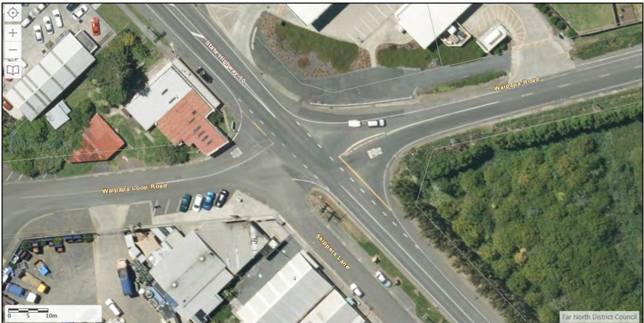
Figure 1-3 Waipapa Road and SH10 Intersection
