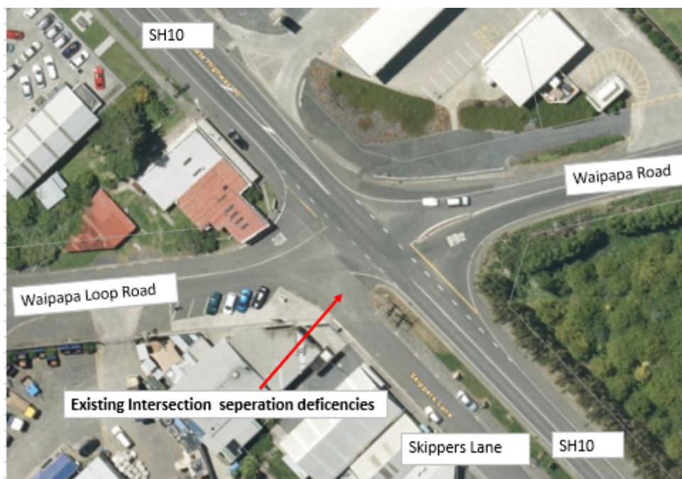
Figure 14: Existing intersection separation deficiencies
