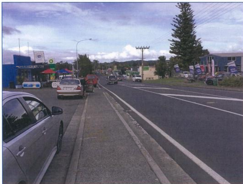
Figure 19: The SH10 north approach, 70 m in advance of the roundabout.
