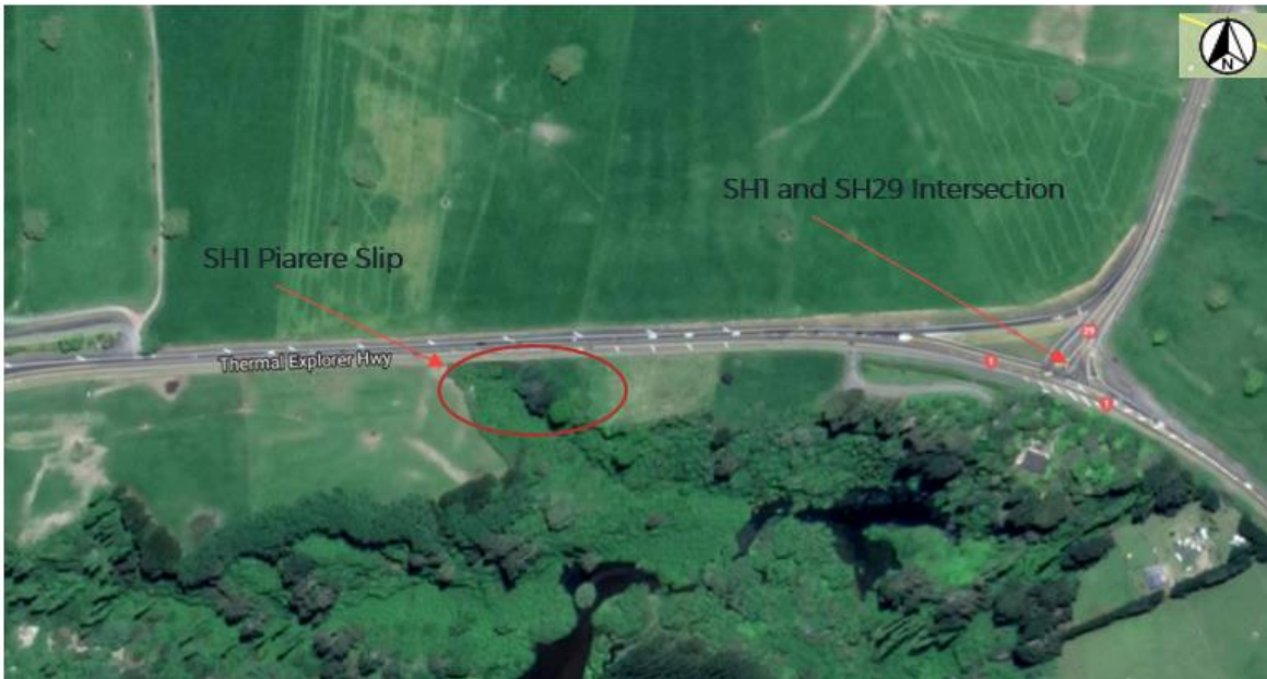
Figure 5.4-1: SH1 Piarere Slip – location of known instability
