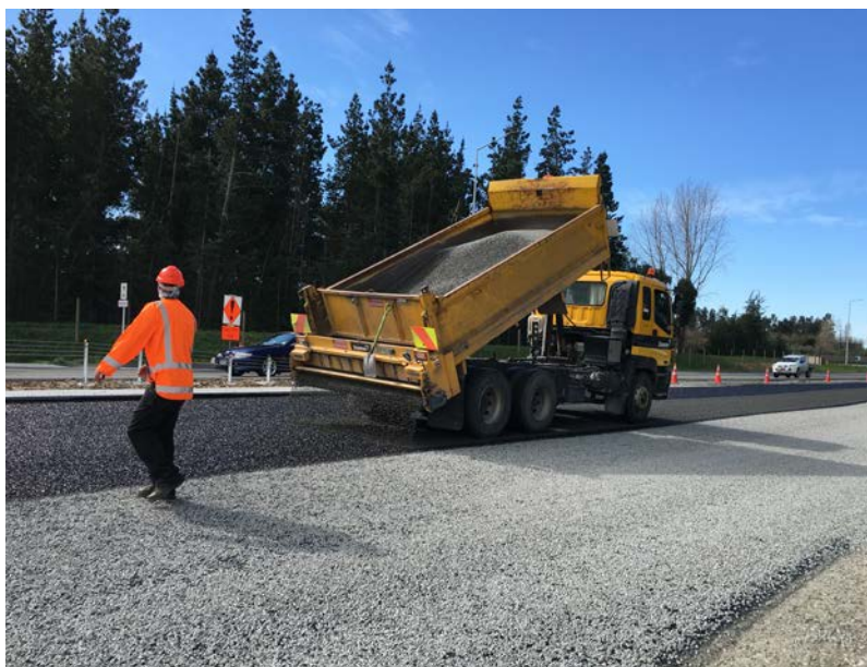
Above: Chipsealing southbound lanes
