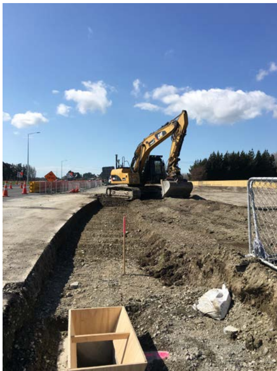
Kerb and channel preparation: Sawyers Arms Roundabout
