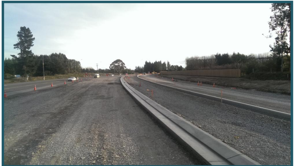
New Concrete Median Island – North of Clearwater Avenue
