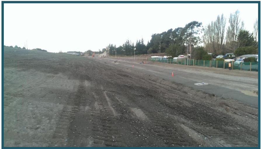
New Greywacke Link Road behind North – South Holiday Park
