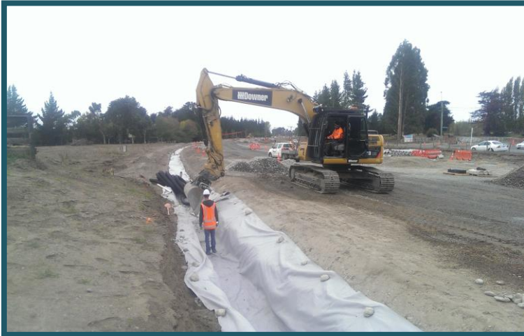
Installing Subsoil Drains 390 Johns Road
