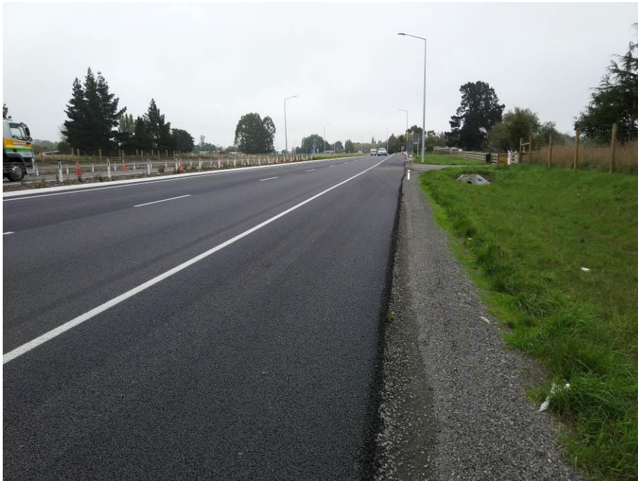
Above: Freshly laid epoxy modified asphalt, south of Clearwater Roundabout.
