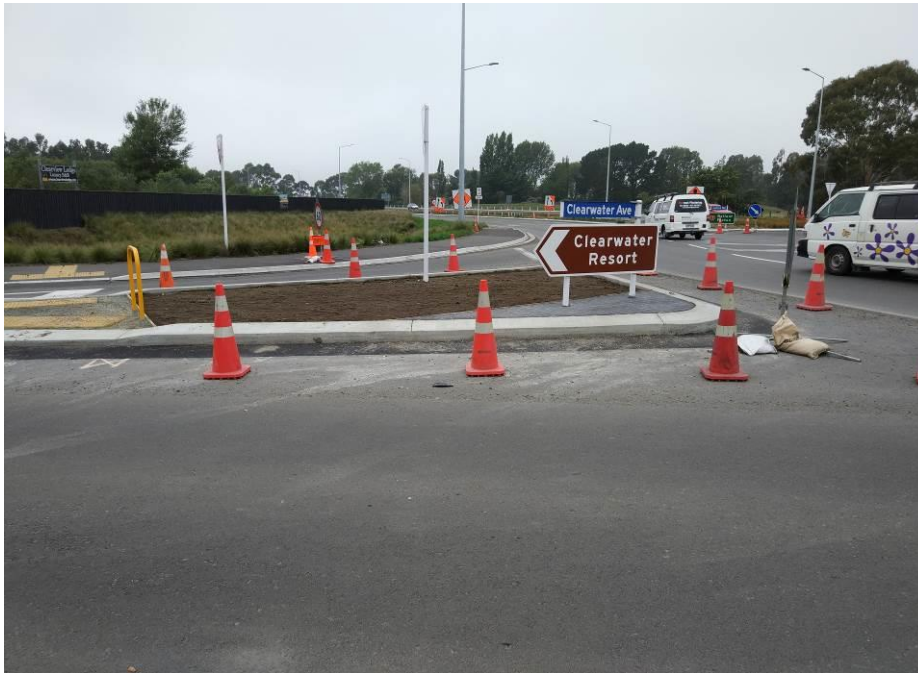
Above: New Clearwater Avenue splitter island
