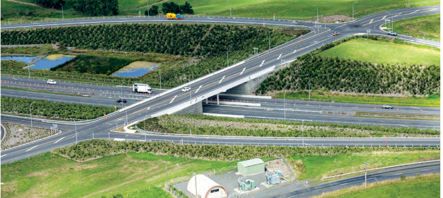
The Te Kauwhata interchange
