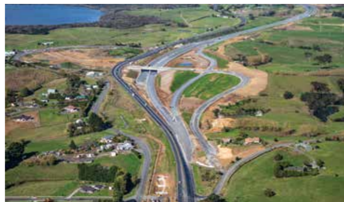
Te Kauwhata interchange looking south
