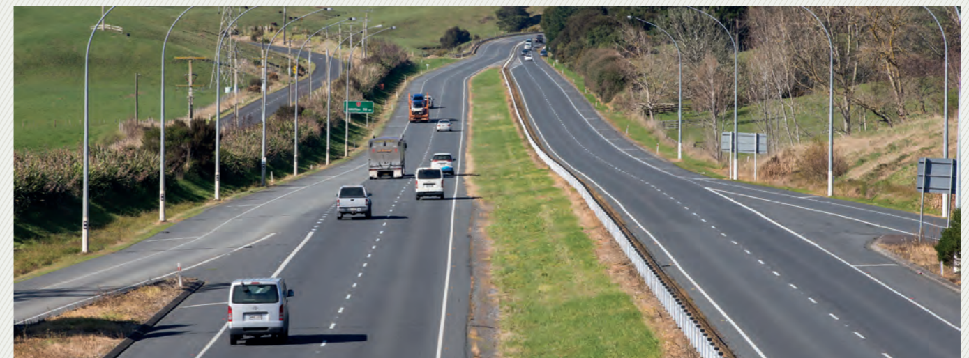
Looking south from Hampton Downs. Work will start on the Longswamp section in October, starting where the project will connect to the current four lanes.
