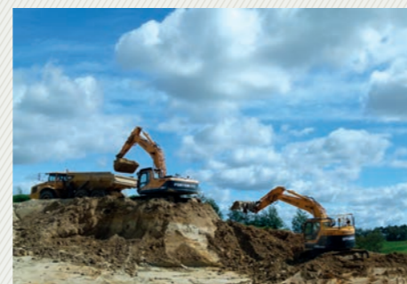
Earthworks at Rangiriri
