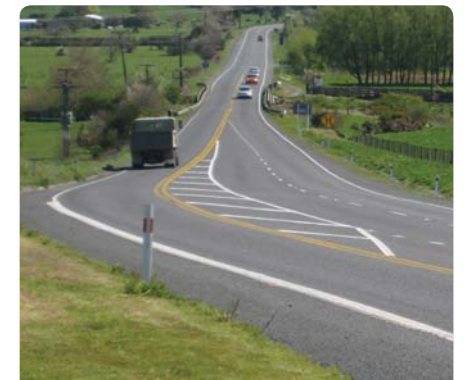
KOPUKU REALIGNMENT. View Over Mangatangi Bridge
