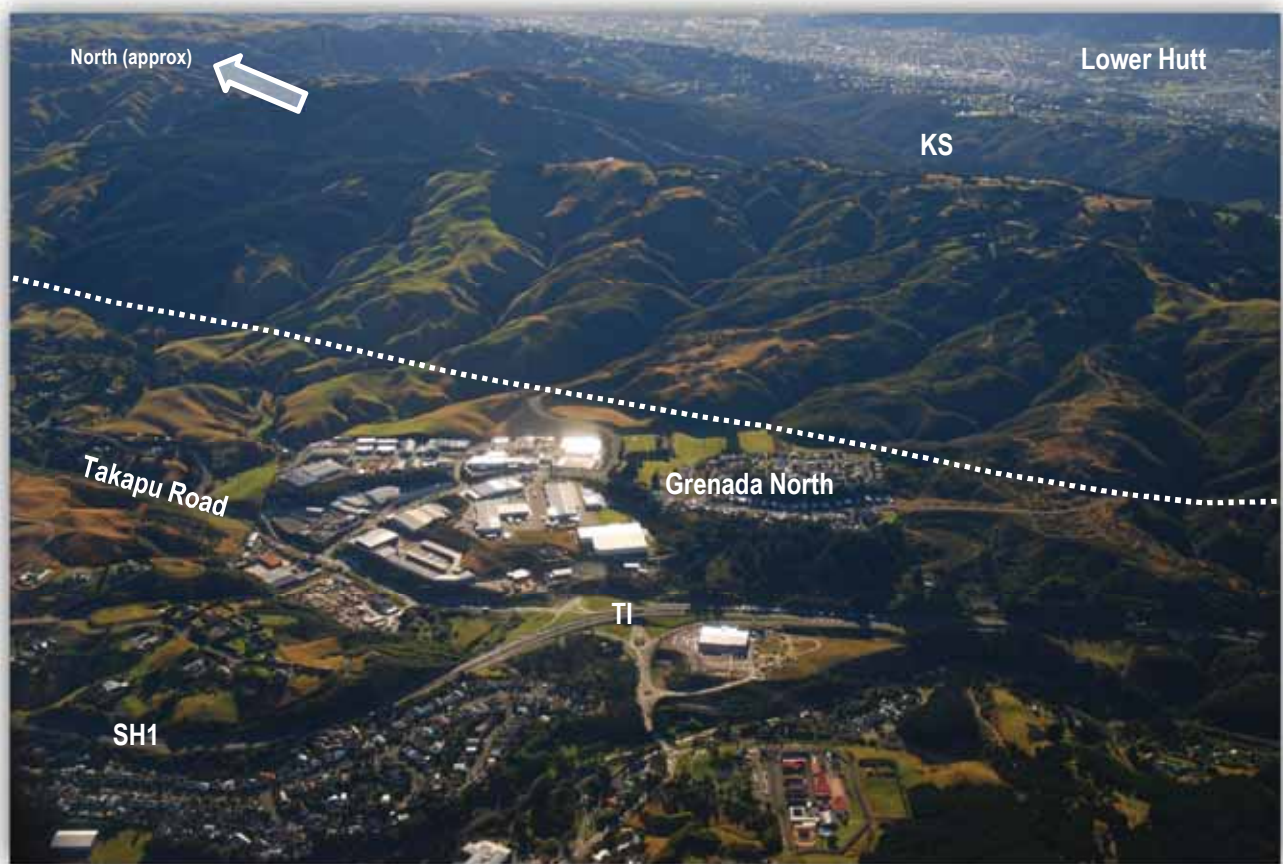
Illustration 5 Oblique aerial photo – Takapu Road
