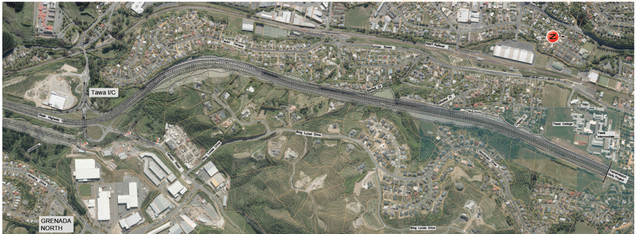
Figure 2p –SH1 Full Widening Between Tawa and Transmission Gully (Adding Additional Lanes on Outside of Existing Carriageway)
